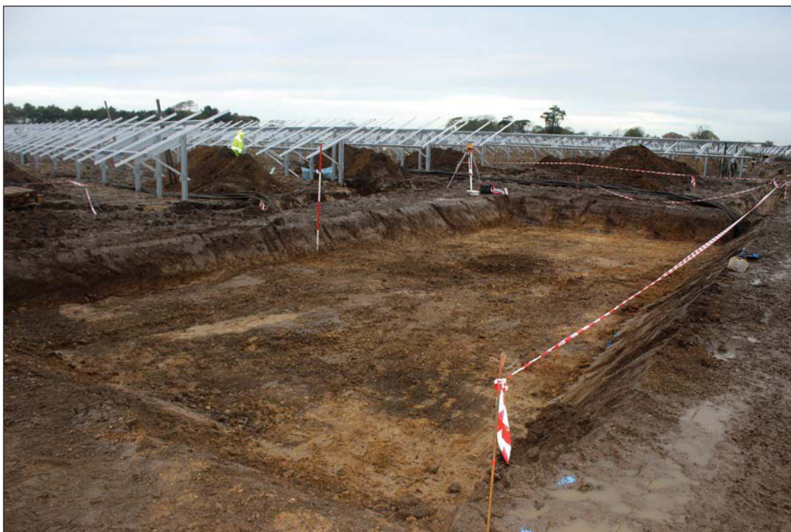
Plate 2. The transformer base, looking north-west, Scale: 2m
