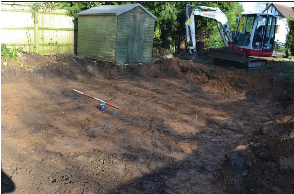
Plate 2. Area of overburden strip looking north east, Scale: 2m.
