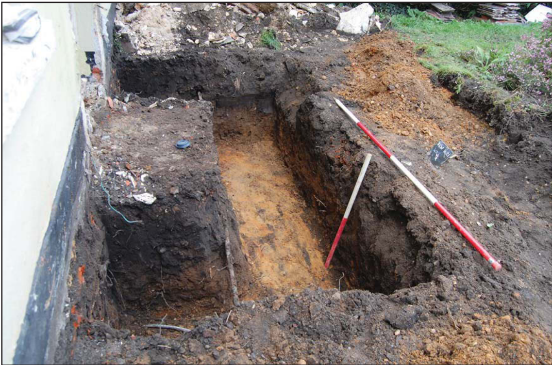
Plate 1. Footing trench for the porch, looking northwest, Scales: 2m and 1m.
