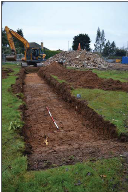
Plate 3. Trench 3, looking north west, Scales: horizontal 2m and 1m, vertical 0.3m.
