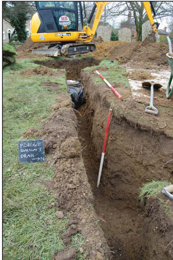
Plate 5. Soakaway 3 drainage pipe trench, looking west, Scales: 2m and 1m.
