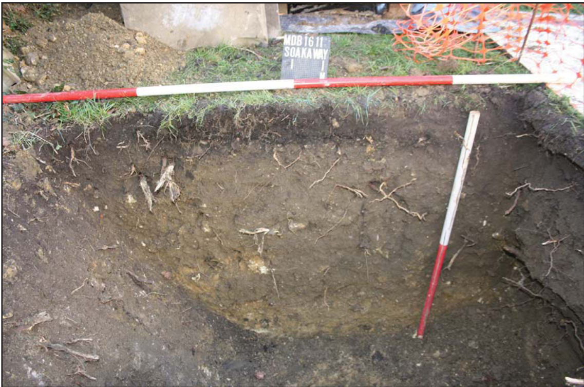
Plate 4. Soakaway 1 section, looking south, Scales: 2m and 1m.
