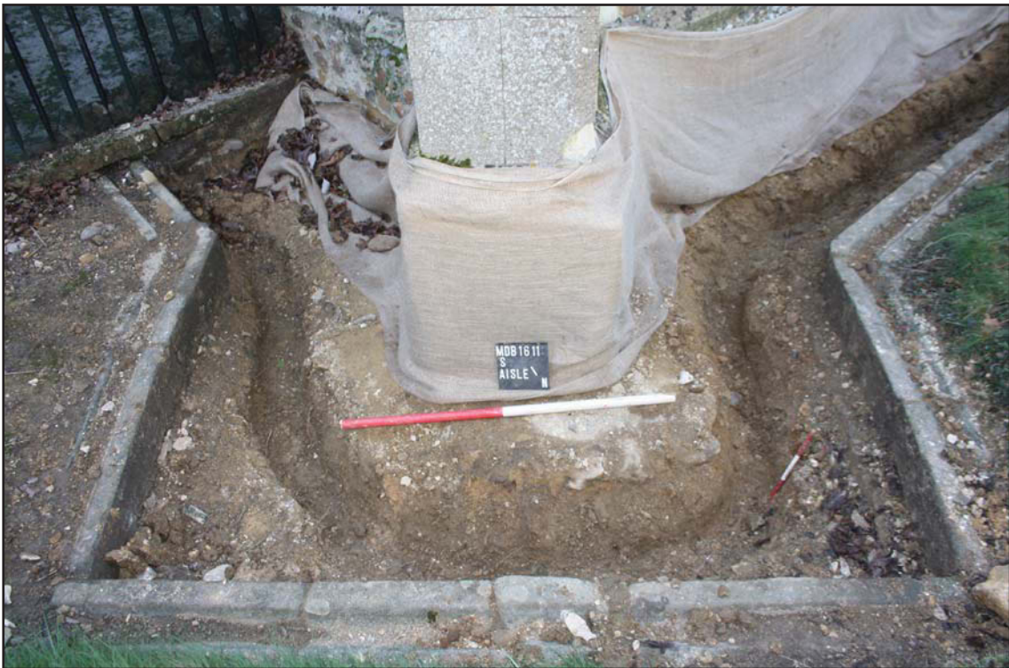
Plate 2. South aisle dry area, looking south-west, Scales: 1m and 0.3m.
