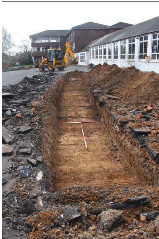
Plate 4. Trench 8, looking South, Scales: 2m, 1m and 0.3m.
