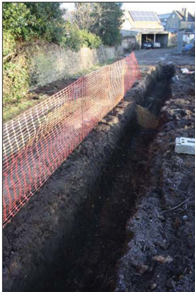
Plate 3. Retaining wall trench looking north.
