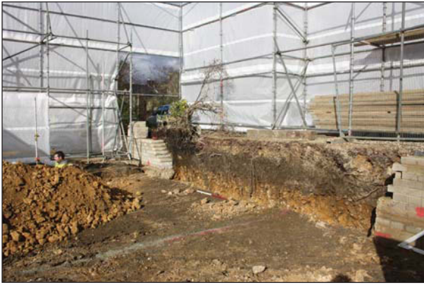
Plate 1. General view of site, looking east.
