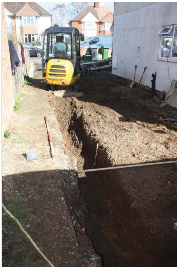
Plate 1. Foundation trench, looking northwest, Scales: horizontal 2m and vertical 0.50m.
