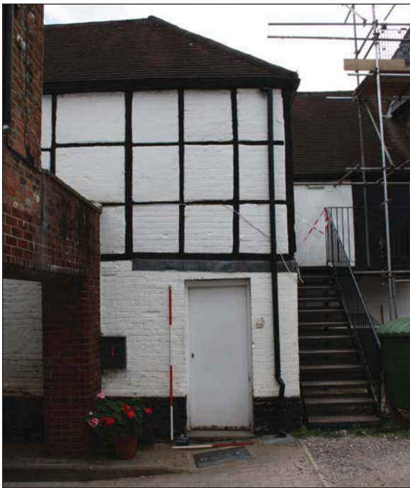
Plate 3. Timber framing, looking north-east
