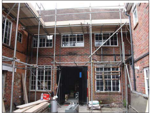
Plate 2. Internal courtyard, looking south-west
