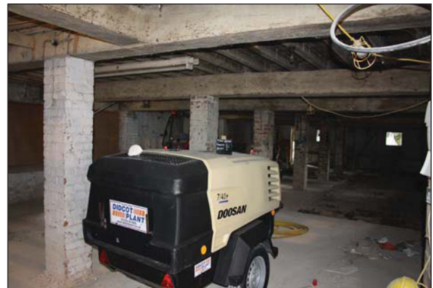
Plate 18. Room 1 looking south-east TMH 15/169
