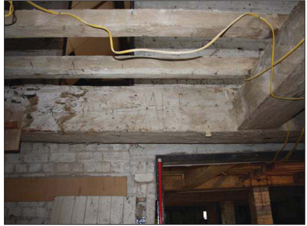
Plate 20. Carpenters' marks, room 2
