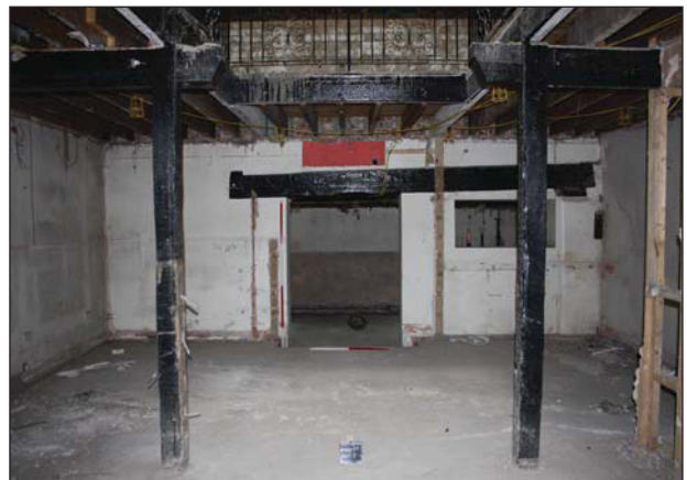
Plate 12. Room 8, looking north-east
