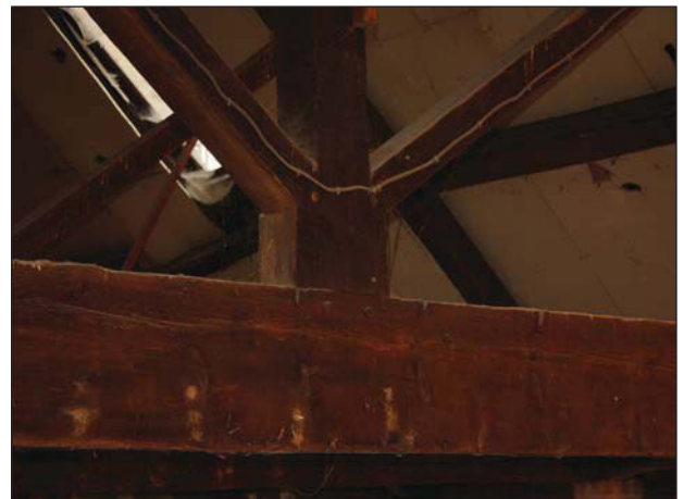
Plate 22. Carpenters' marks, room 14
