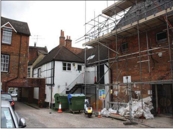
Plate 1. Timber framed range, looking north
