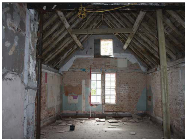
Plate 29. Room 11, gable end, looking south-east
