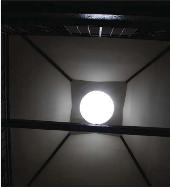
Plate 13. Room 8, roof space
