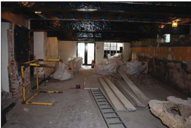
Plate 25. Room 6, looking north-west
