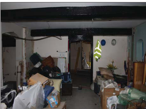
Plate 4. Room 4, Door, looking south
