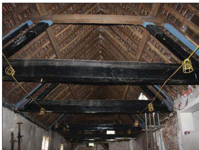
Plate 28. Room 10, roof truss
