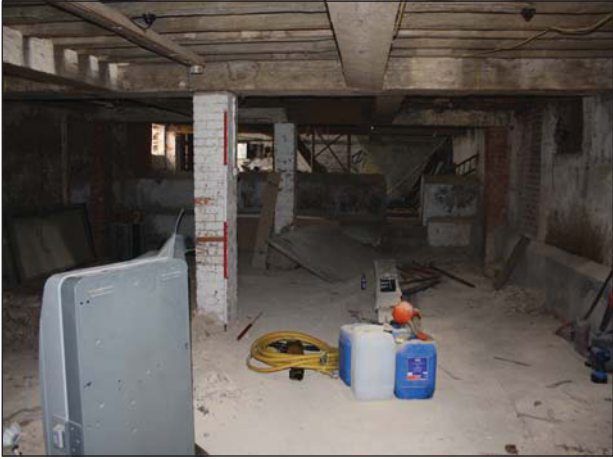
Plate 19. Room 2, looking north-east
