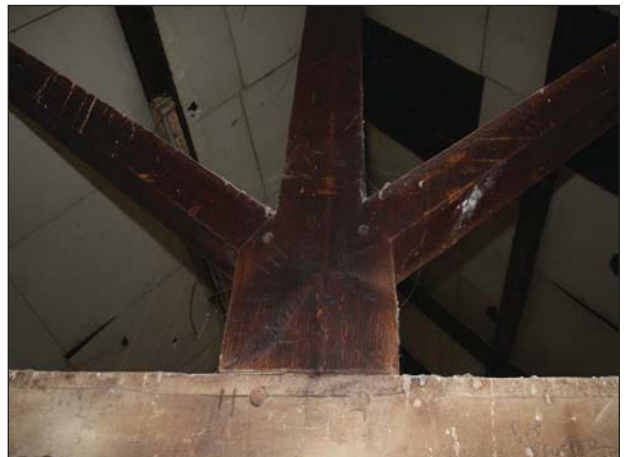
Plate 24. Carpenters' marks, room 13
