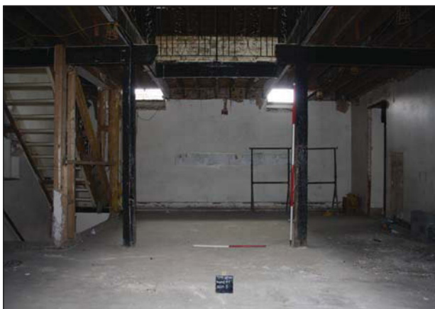
Plate 11. Room 8, looking south-west
