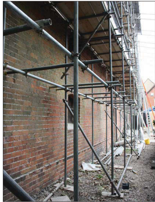
Plate 17. Rear range looking north-west
