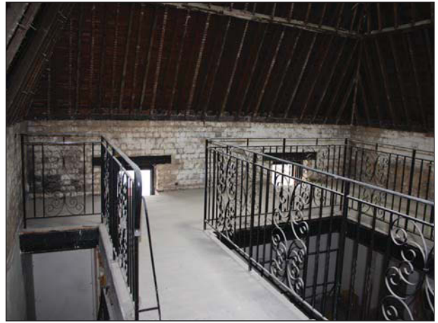
Plate 14. Room 9, looking north-west
