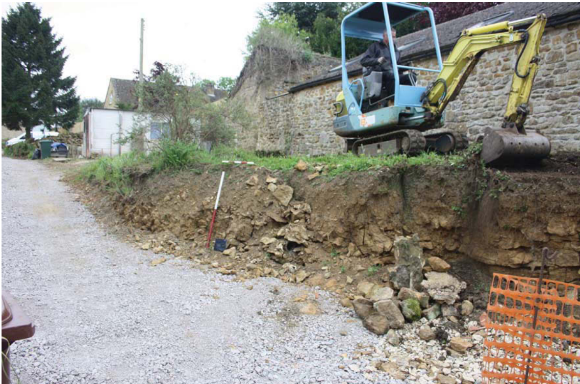
Plate 1. Exposed section of site makeup, looking south, Scales: 1m and 0.5m.
