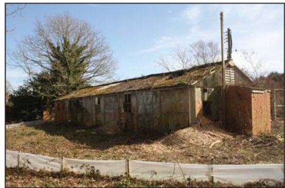
Plate 4. Building A, looking East
