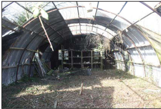
Plate 5. Interior, building B, looking NNW
