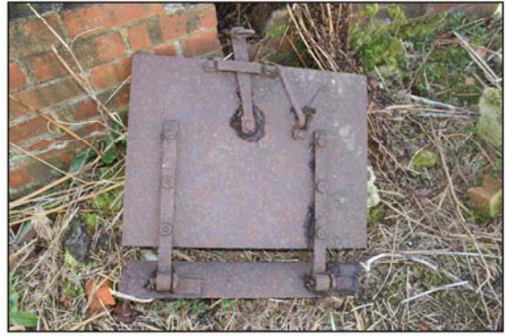
Plate 2. Detail of incinerator door, building L
