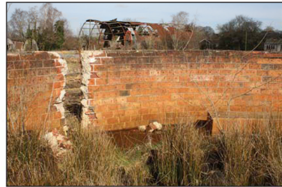
Plate 6. Inside of structure R
