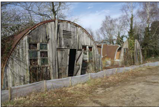
Plate 3. Buildings C and B, looking NNW
