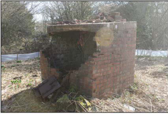
Plate 1. Building L from the north-west.
