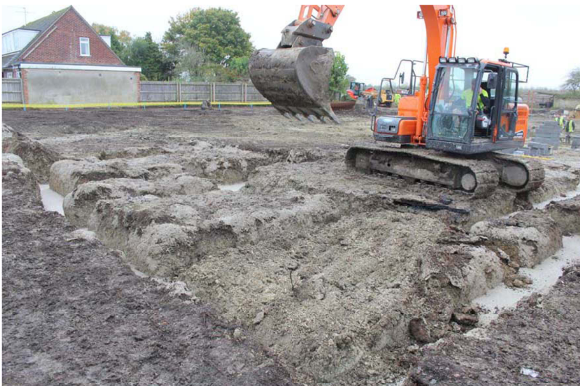
Plate 2. Plot 1, stripping after concreting of footing, looking south east.
