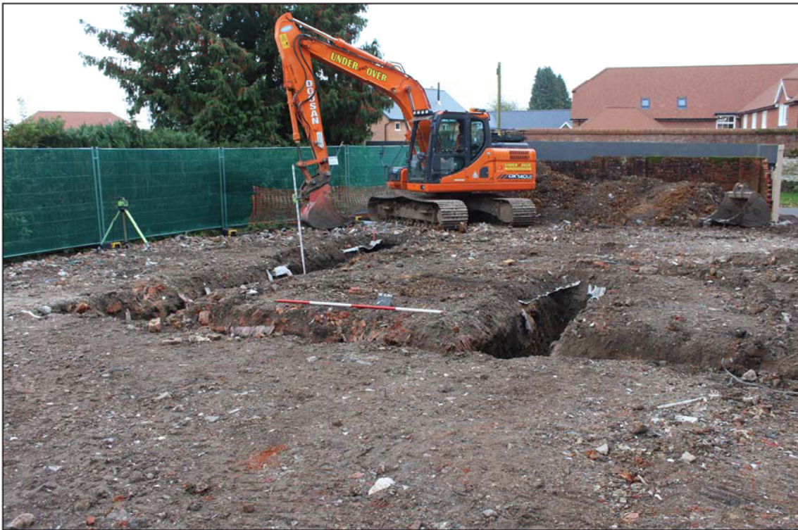
Plate 1. Plot 1 under excavation, looking south east, Scale: 2m.
