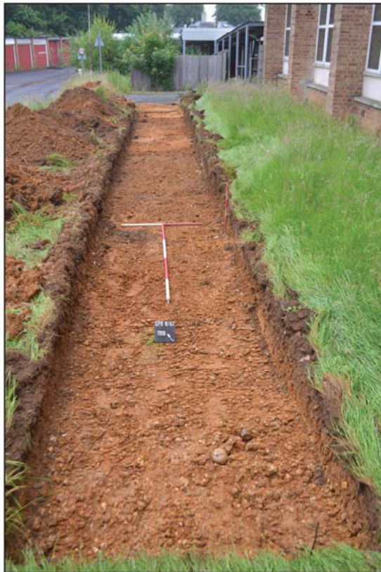
Plate 4. Trench 19, looking north east, Scales: horizontal 2m and 1m, vertical 0.5m.
