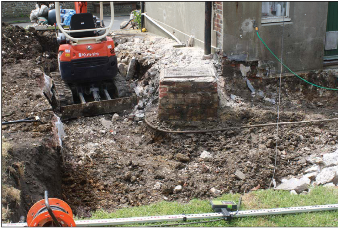
Plate 1. General view of site looking south.
