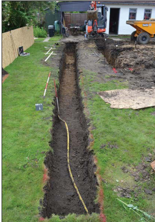
Plate 1. Boundary wall footing, looking south, Scales: 2m and 1m.
