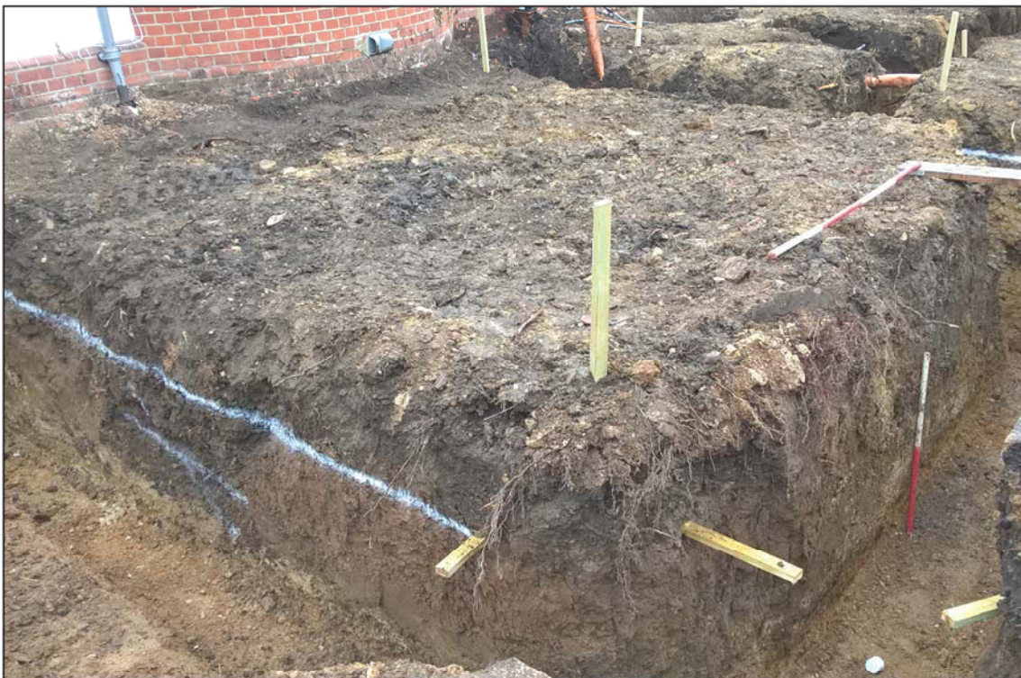
Plate 2. Footing sections, looking east, Scales: 2m and 1m.
