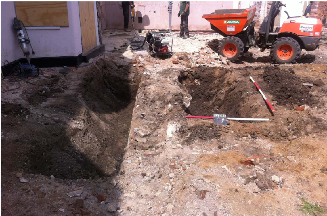
Plate 2. Excavation showing footing, looking north, Scales: 2m and 1m.
