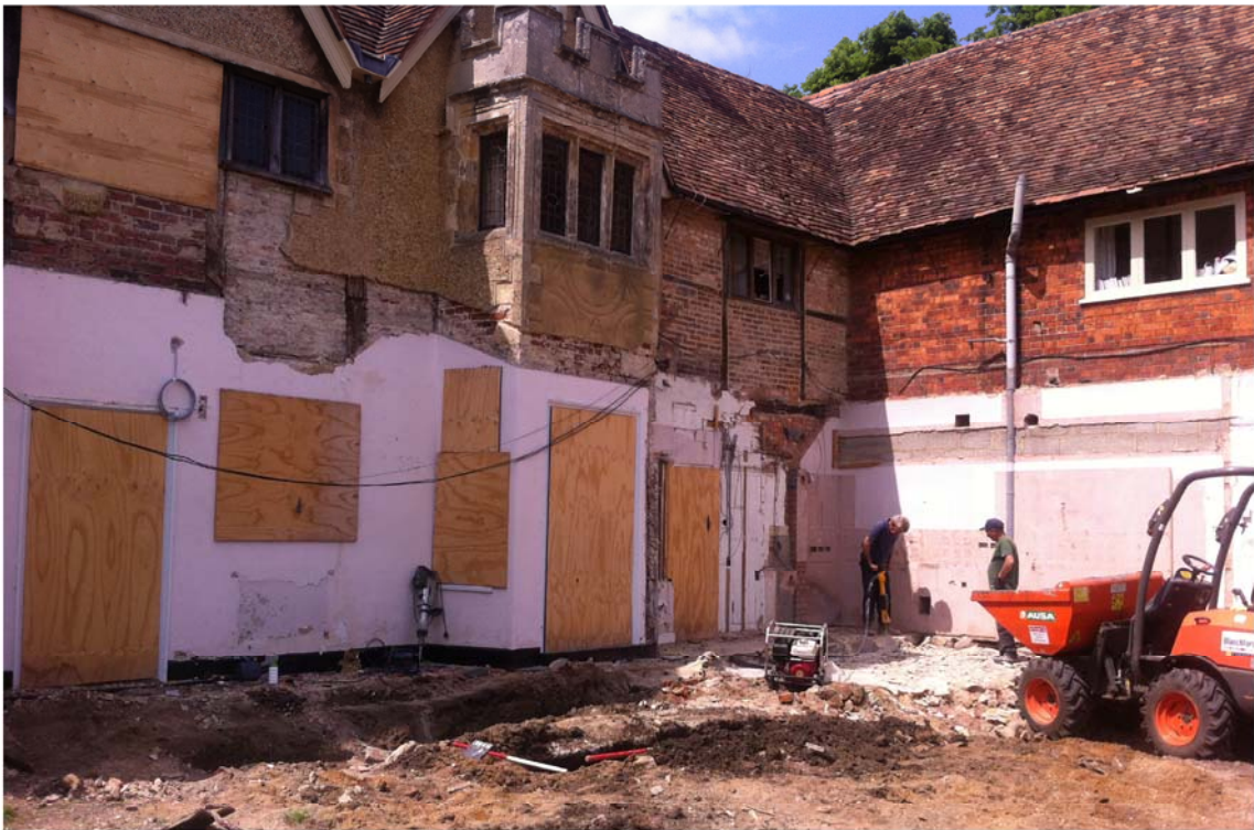
Plate 1. Area of excavation, looking north west.
