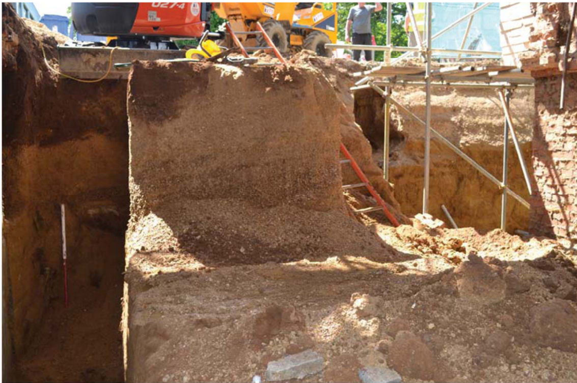
Plate 1. Interior excavation, looking south, Scale: 1m.
