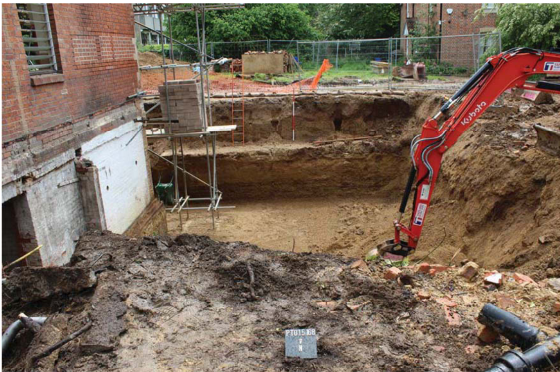
Plate 2. Exterior excavation, looking south, Scale: 2m.
