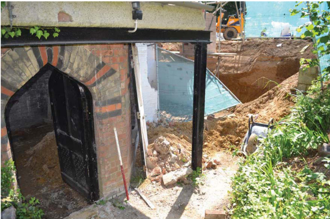
Plate 4. Retained cellar door, looking east, Scale: 1m.
