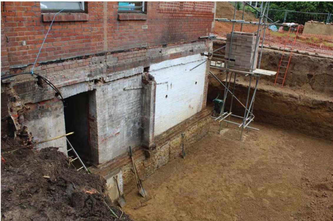
Plate 3. Exterior excavation, completed, looking southeast.
