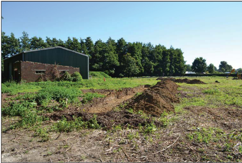
Plate 2. General view of trenches 5 and 4 during trenching, looking north east
