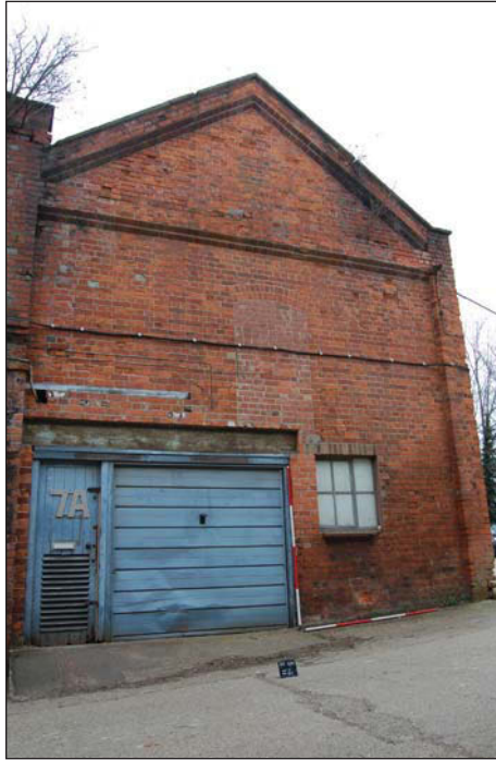
Plate 33. Exterior, Unit 7a, looking east north east, Scales: 2m.
