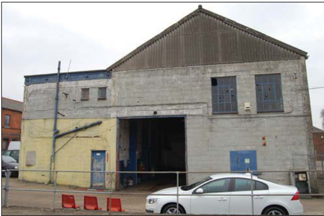
Plate 19. Exterior, Unit 3, looking west, Scales 2m.
