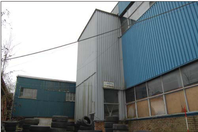
Plate 43. Exterior, Unit 9, looking north west, Scale: 2m.
