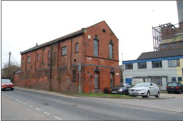
Plate 1. Site view, looking south east, Scales: 2m and 1m.
