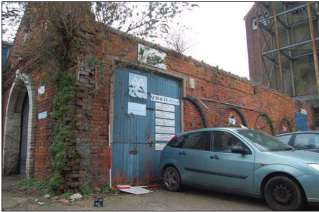
Plate 41. Exterior, Unit 8, looking south west, Scales: 2m.
