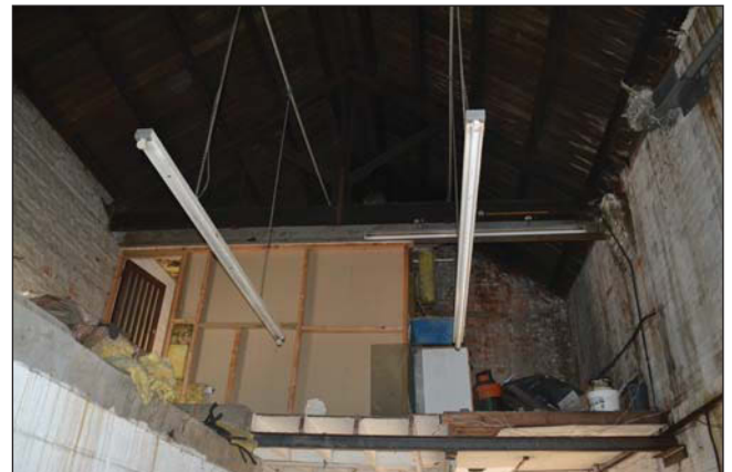
Plate 36. Interior, Unit 7d ground floor, looking north, Scales: 2m.
