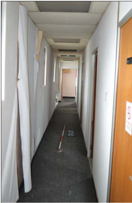
Plate 11. Interior, Counting House first floor corridor, looking east, Scale: 2m.
