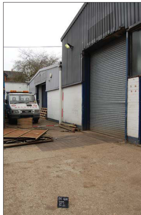
Plate 16. Exterior, Unit 1, looking west, Scales: 2m.
