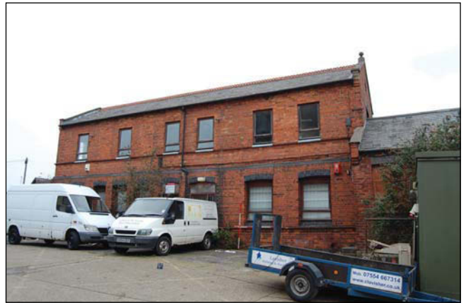
Plate 4. Exterior, The Counting House, looking north, Scales: 2m and 1m.
