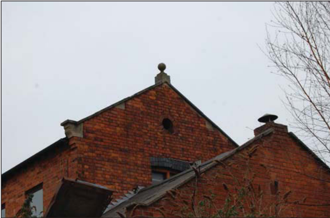
Plate 5. Exterior, roof gable detail, looking north west.
