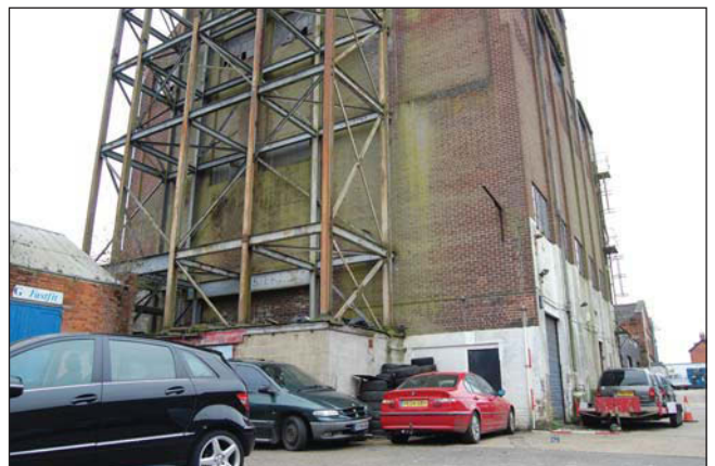
Plate 24. Exterior, Unit 7 lower, looking north east, Scales: 2m.
