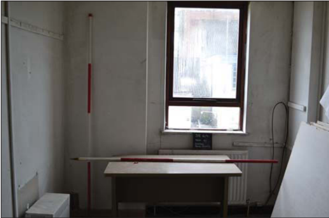
Plate 13. Interior, Counting House first floor, room 7, looking south south east, Scales: 2m.
