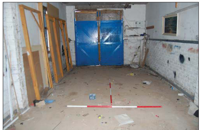
Plate 48. Interior, Unit 12, looking east, Scales: 2m.
