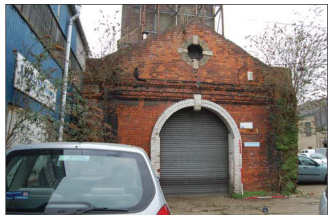
Plate 40. Exterior, Unit 8, looking west, Scales: 2m.
