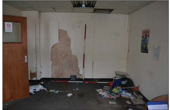
Plate 6. Interior, room 1, Scales: 2m and 1m.
