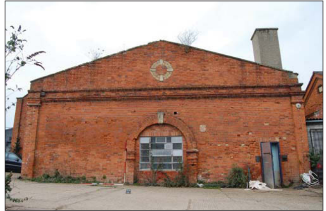
Plate 34. Exterior, Unit 7a, looking north, Scales: 2m.
