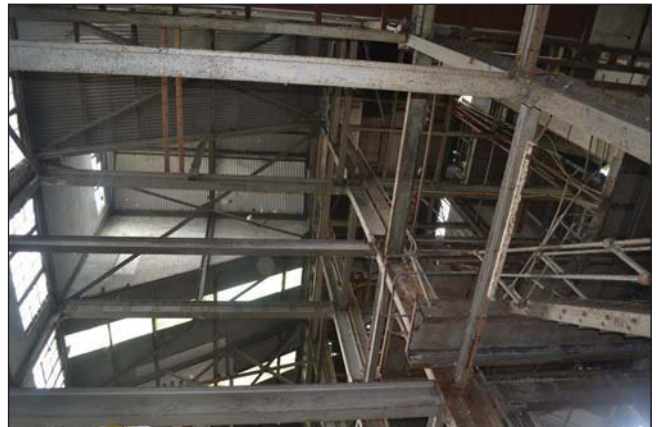
Plate 28. Interior, Unit 7 roof structure.
