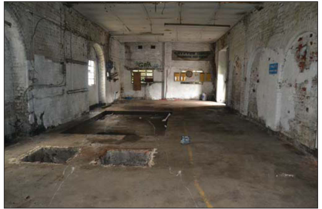
Plate 42. Interior, Unit 8, looking east, Scales: 2m.
