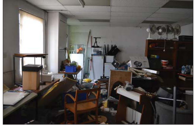
Plate 10. Interior, Counting House Ground floor, room 5, looking west, Scale: 2m.
