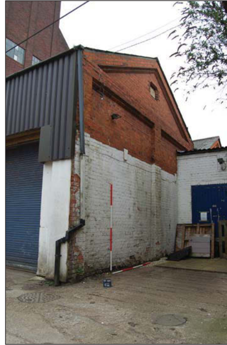
Plate 30. Exterior, Unit 7 oblique end gable, looking south south west, Scales: 2m.
