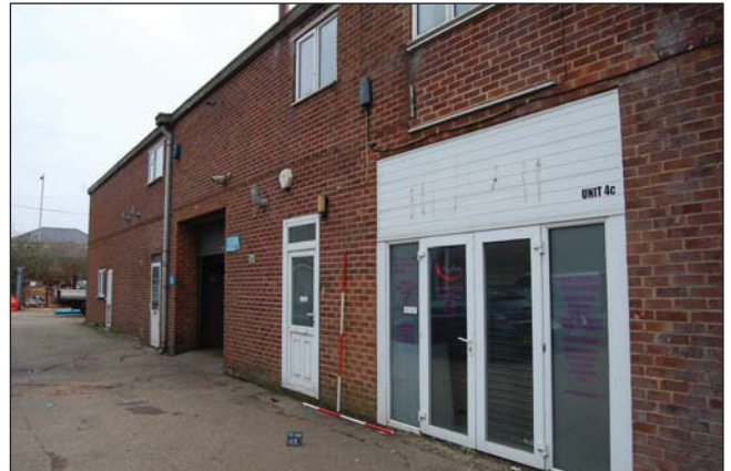
Plate 22. Exterior, Unit 4, looking north east, Scales: 2m.
