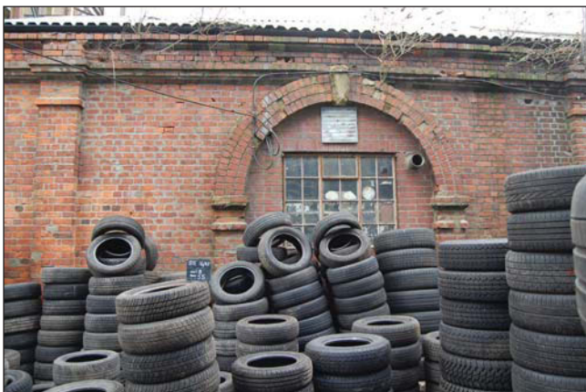
Plate 39. Exterior, Unit 8 window detail, looking north.
