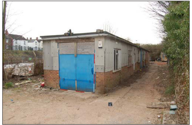
Plate 46. Exterior, Unit 12, looking south west, Scales: 2m.
