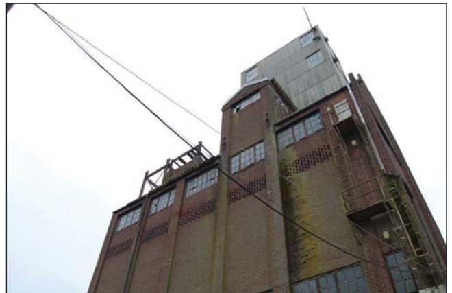
Plate 26. Exterior, Unit 7 upper, looking south.
