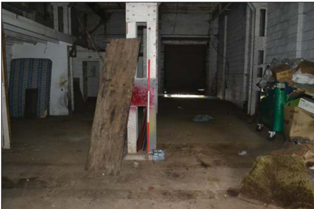
Plate 27. Interior, Unit 7, looking north, Scale: 2m.
