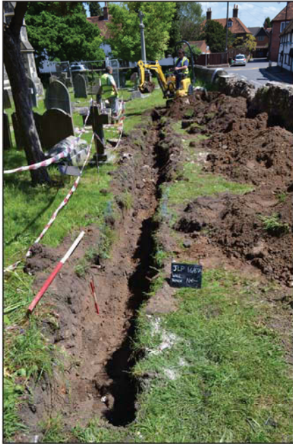
Plate 1. Footing Trench, looking East, Scales: Horizontal 1m and Vertical 0.30m.
