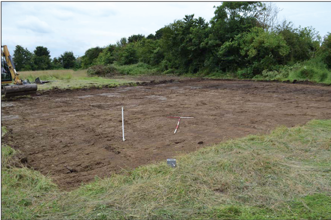
Plate 1. Topsoil strip, looking south west, Scales: 2m and 1m.
