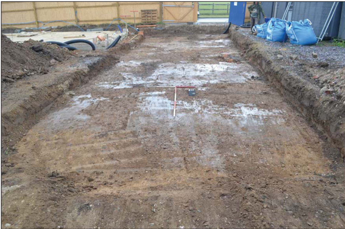
Plate 3. Access road, looking west, Scales: 1m and 2m.
