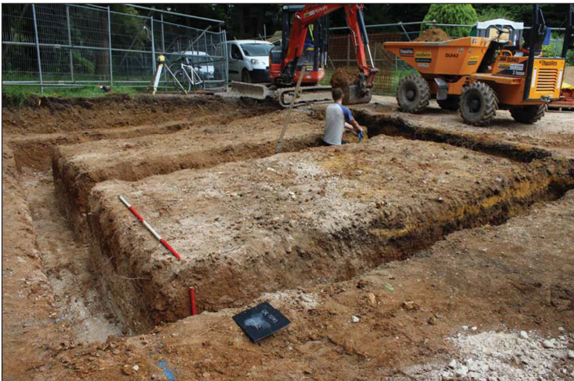
Plate 4. Garage footing trenches, looking SW, Scales: 2m and 1m.
