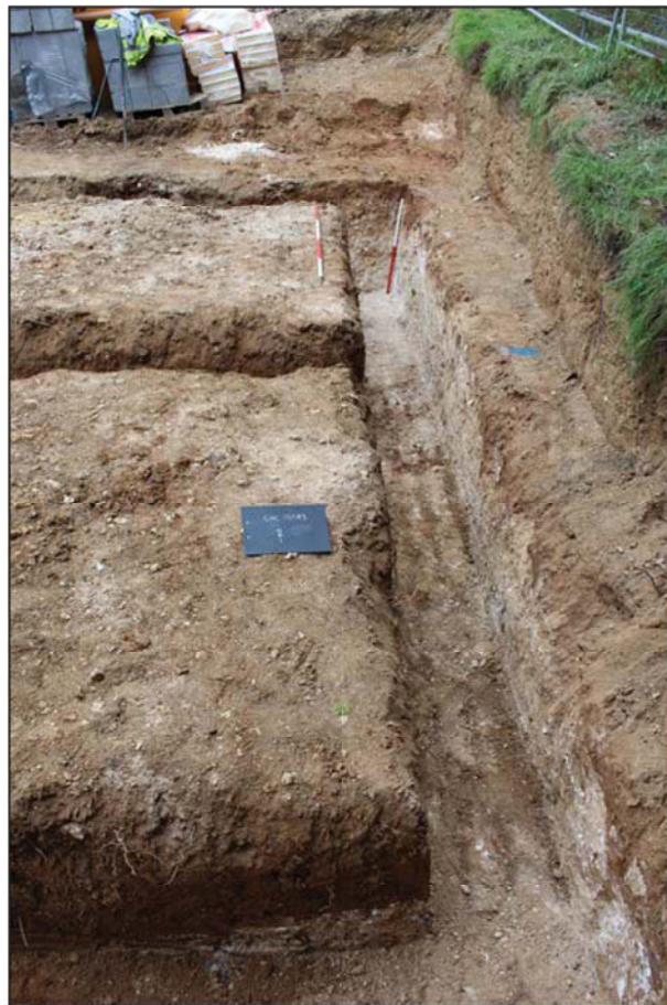
Plate 2. Garage footing trenches, looking N, Scales: 1m and 2m.
