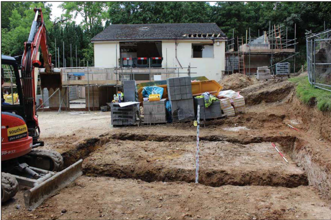
Plate 3. Site, looking N, Scales: 2m and 1m.
