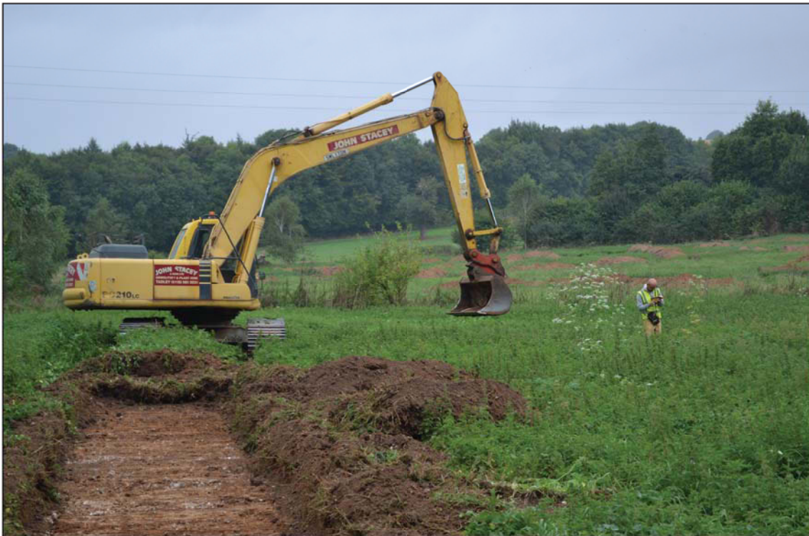
Plate 6. General view of site looking west.
