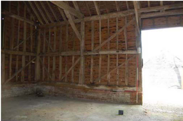
Plate 23. Southwest barn, timber frame detail, looking north, Scales: 2m and 1m..
