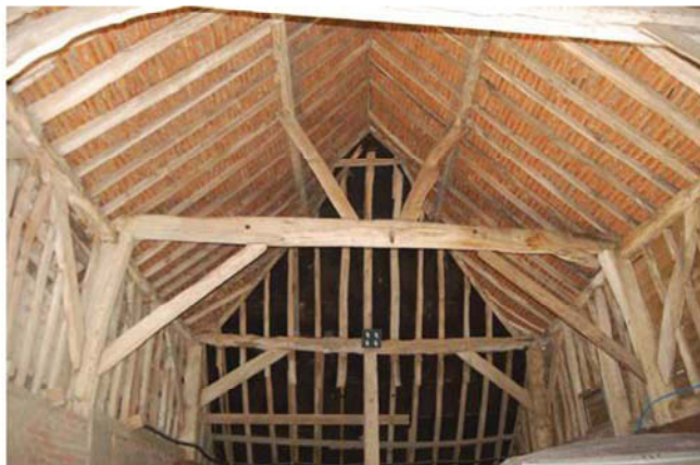
Plate 8. Northwest barn, trusses at west end, looking west.
