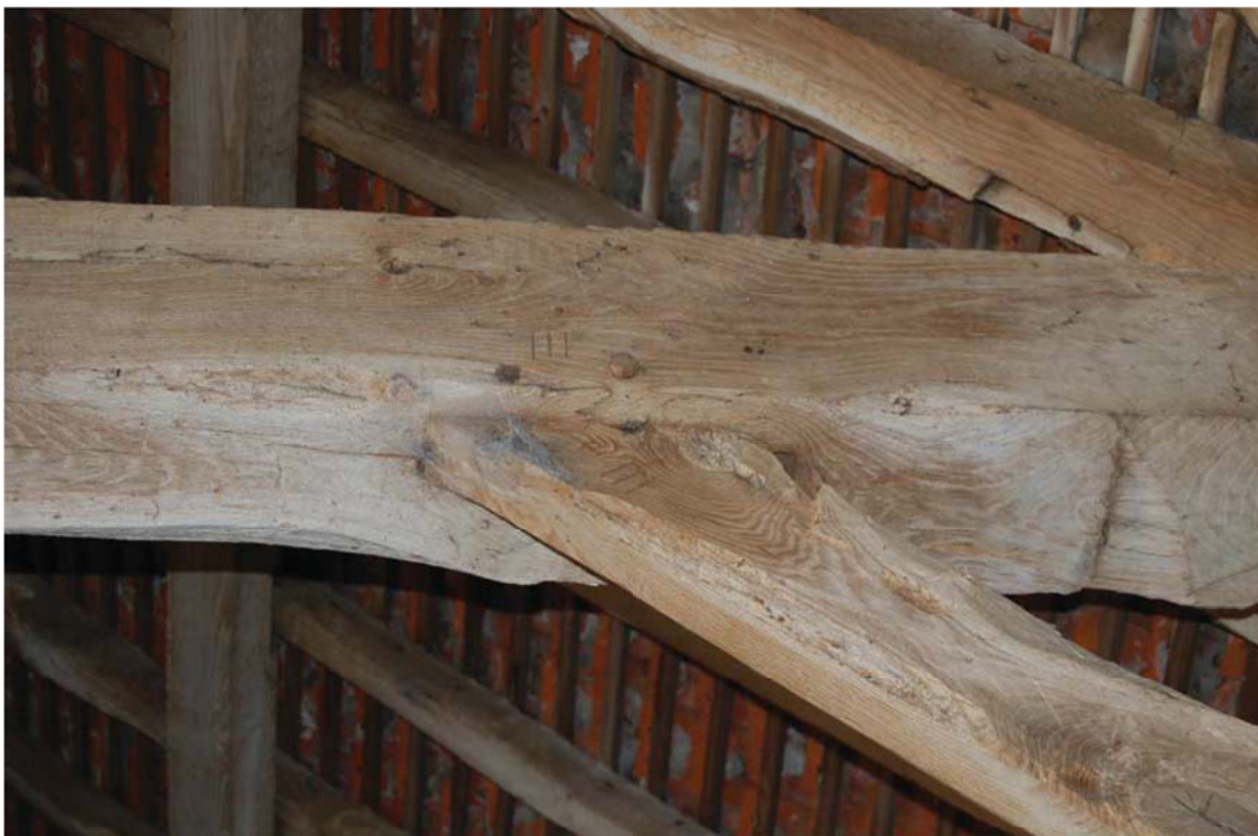
Plate 26. Southwest barn, carpenters mark 'III', looking east.
