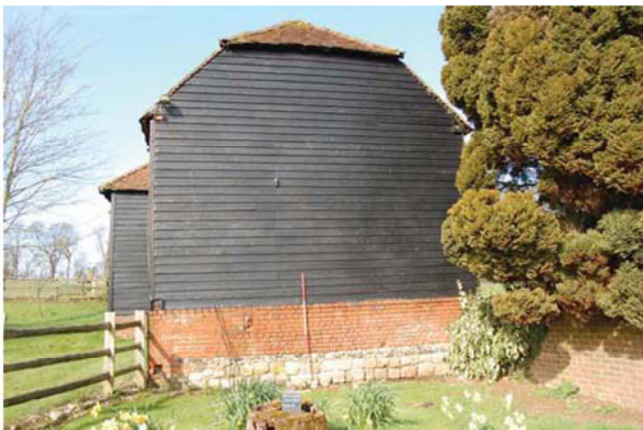
Plate 19. Southwest barn, east elevation, looking west, Scales: 2m and 1m..
