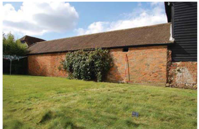
Plate 16. Rear of stable block, looking southwest, Scales: 2m and 1m.
