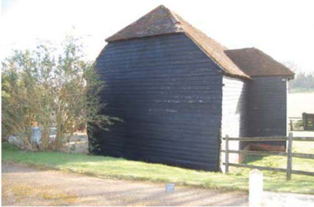
Plate 21. Southwest barn, west and south elevation, looking east.
