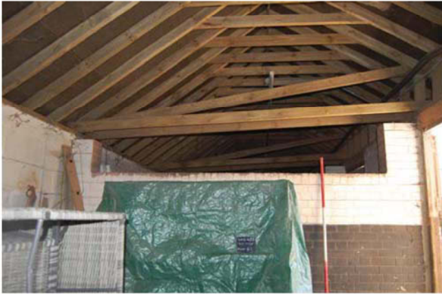
Plate 17. Interior of stables and roof detail, looking south, Scales: 2m.
