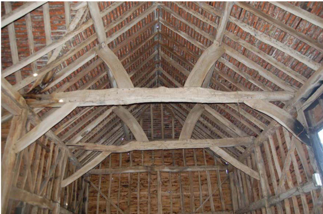
Plate 25. Southwest barn, detail of trusses, looking west.
