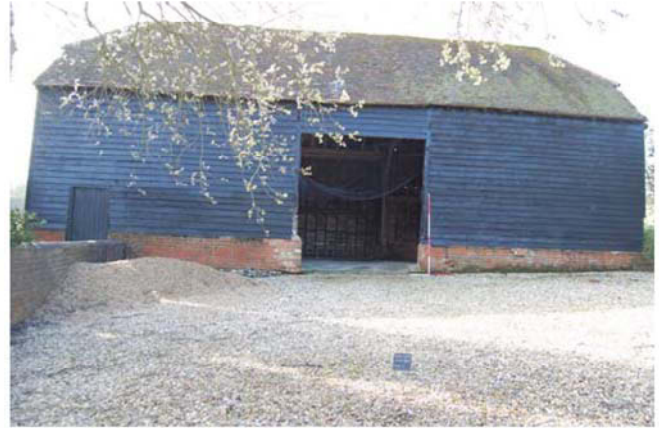
Plate 18. Southwest barn, north elevation, looking south, Scales: 2m and 1m.
