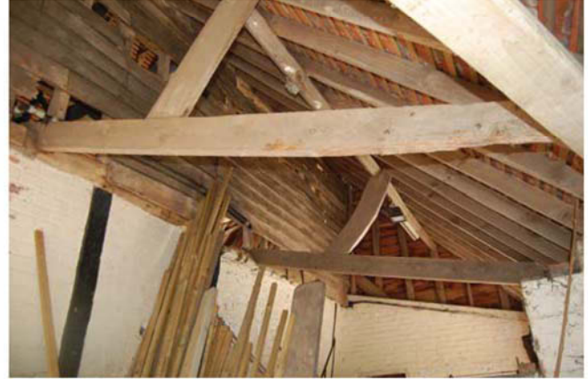
Plate 14. Stables, roof detail, looking northeast.
