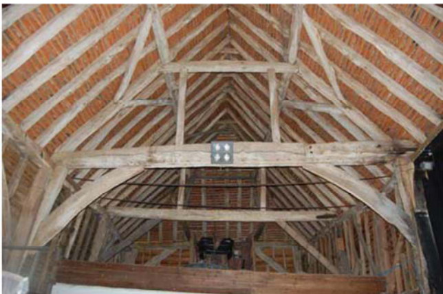
Plate 7. Northwest barn, trusses at east end, looking east.
