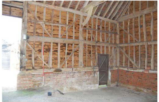
Plate 24. Southwest barn, door inserted in north wall, looking north, Scales: 2m and 1m.
