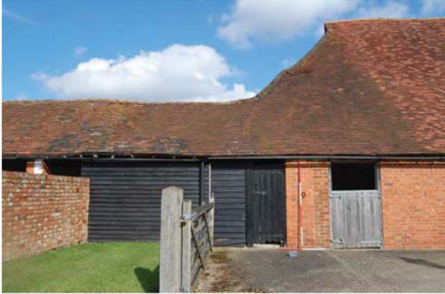
Plate 13. Store and stables, looking north, Scales: 2m and 1m.
