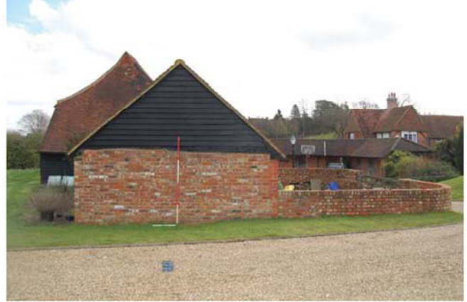
Plate 10. West wall of Cart-shed, looking east, Scales: 2m and 1m.
