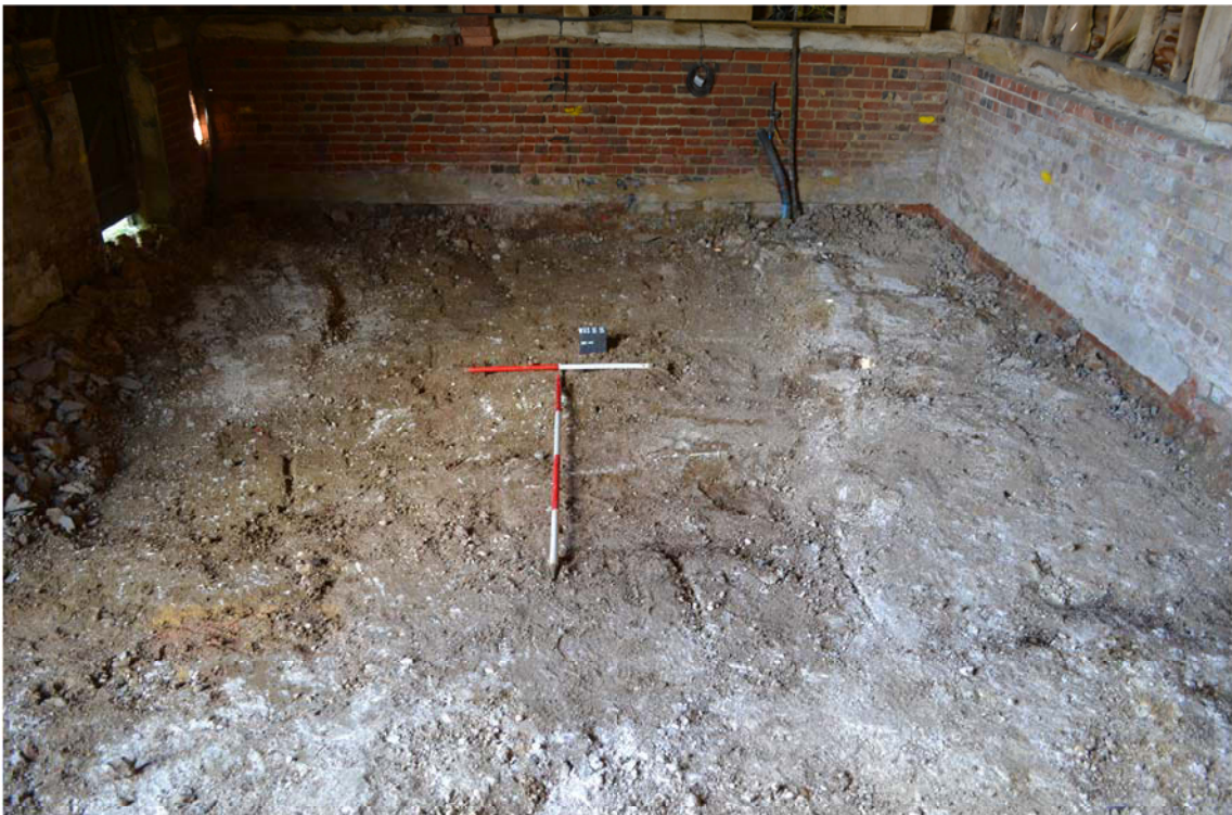
Plate 2. Western side after ground reduction, looking west, Scales: 2m and 1m.
