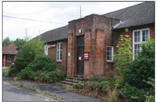
Plate 24. Oblique view of Q4 main entrance, looking southeast.
