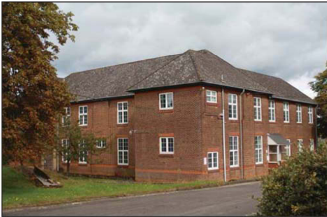
Plate 9. Oblique of Q3, looking northeast.
