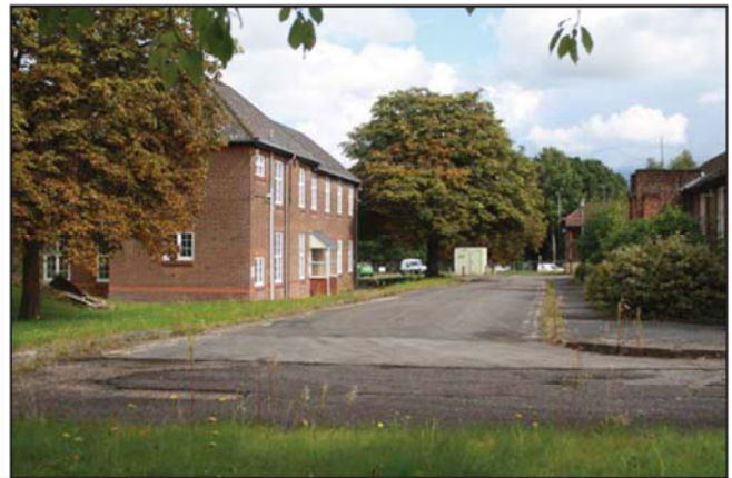
Plate 4. View down road showing Q3 and Q4, looking east.
