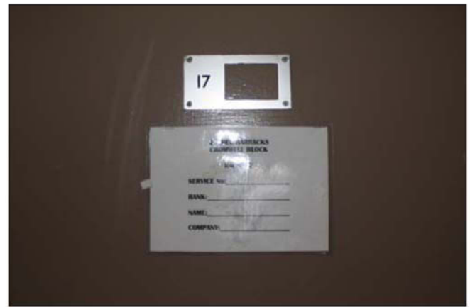
Plate 46. Q8, door label detail, looking southwest.
