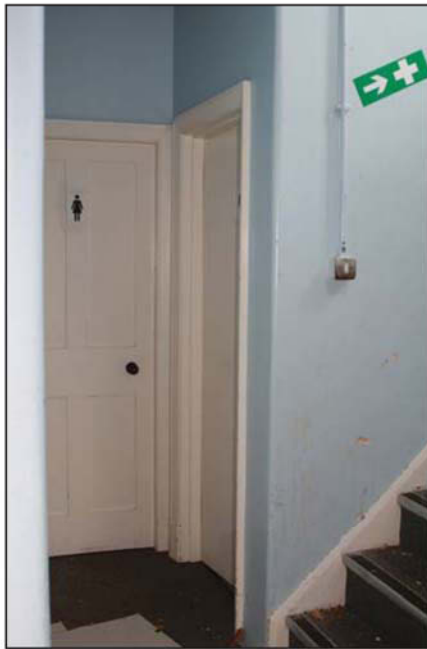
Plate 19. Q3, an original door, looking northeast.
