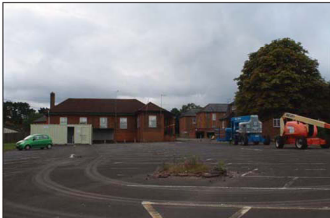
Plate 5. Across car park to Q4 and Q5, looking south-southwest.
