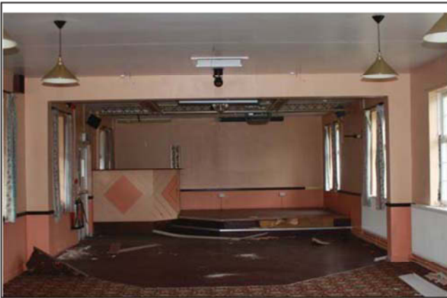
Plate 35. Q5, Lounge, looking north.
