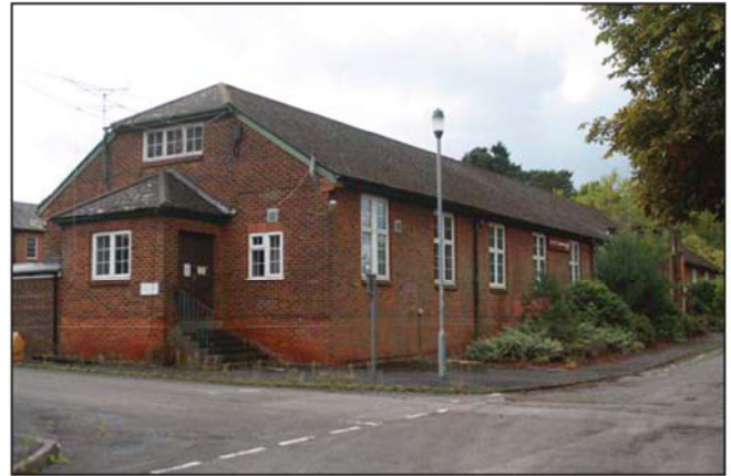
Plate 22. Oblique view of Q4, west end, looking southwest.
