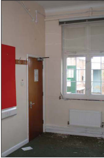
Plate 13. Q3, view to window and door of G.05, looking northeast.
