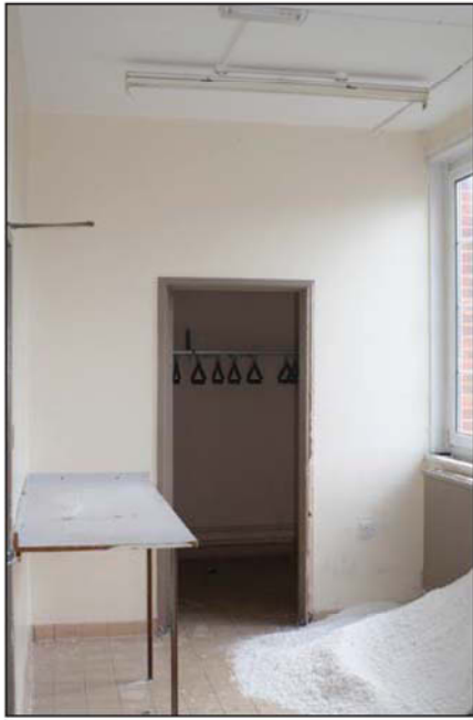
Plate 47. Q8, view to drying room, looking southeast.
