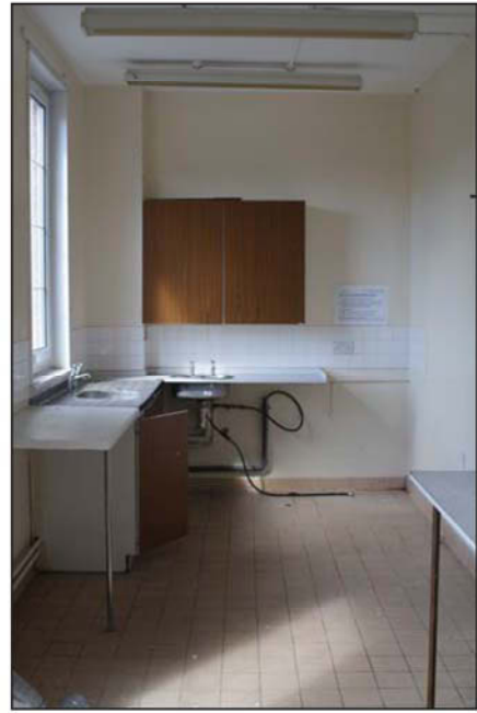
Plate 48. Q8, utility room, looking northwest.
