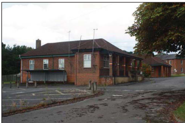
Plate 31. Oblique of Q5, looking southeast.
