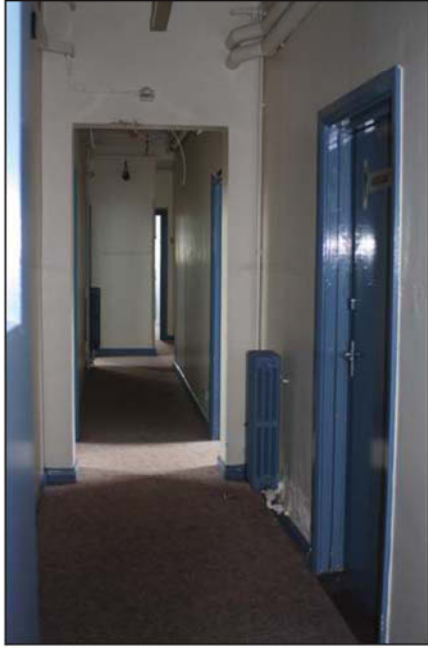
Plate 43. Q6, view along corridor, looking east.
