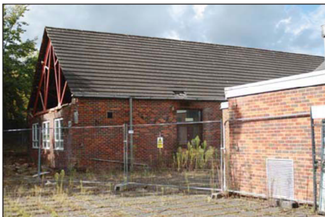
Plate 25. Oblique of Q4SS showing truss detail, looking northwest.
