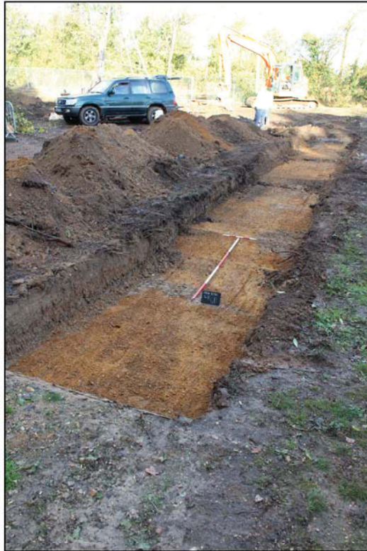
Plate 3. Trench 4, looking north west, Scales: 2m and 0.5m.
