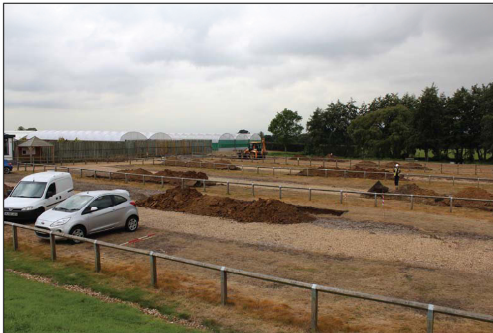
Plate 6. General view of site, looking north east.
