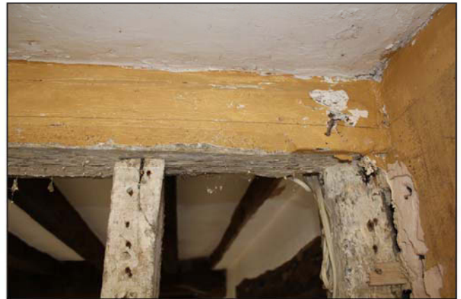
Plate 6. Beam chamfer stop, looking North.
