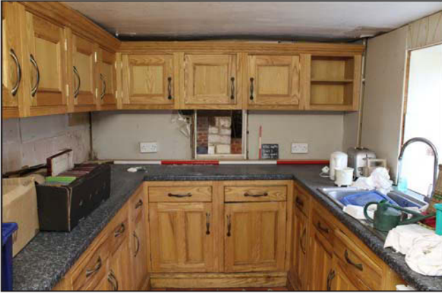
Plate 1. Existing wall, looking South, Scales: 2m and 0.3m.
