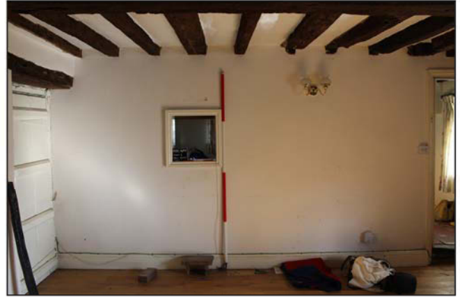
Plate 2. Existing wall, looking North, Scales: 2m and 0.3m.
