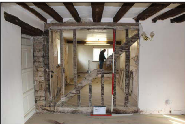
Plate 5. Exposed timber wall, looking North, Scales: 2m and 1m.
