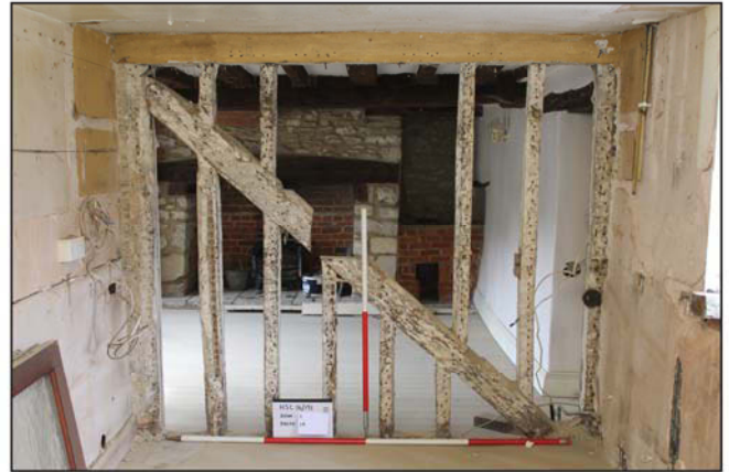
Plate 4. Exposed timber wall looking South, Scales: 2m and 1m.
