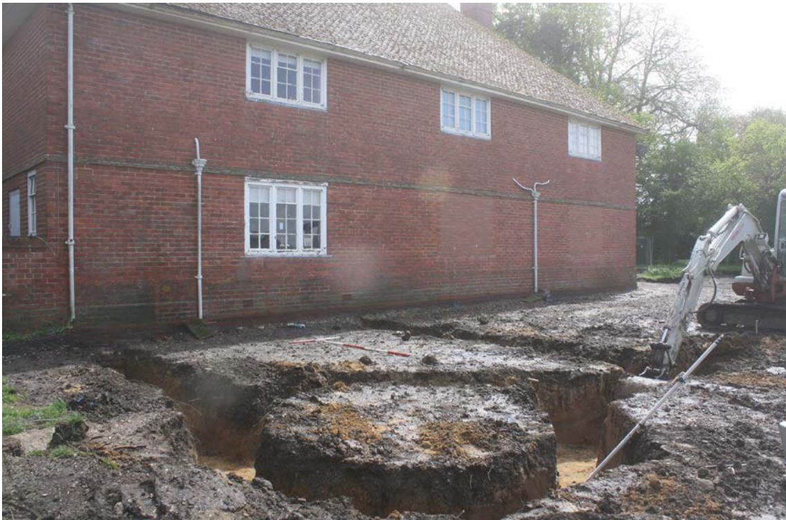
Plate 1. View over footings, looking south east, Scales: 2m and 1m.
