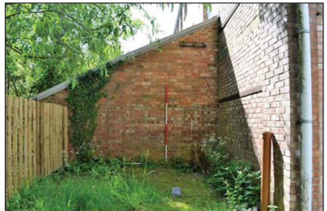
Plate 4. Exterior, rear extension, looking southeast, Scales: 2m and 1m.
