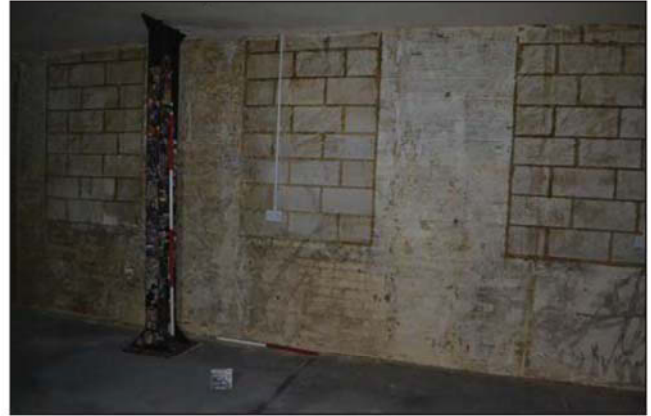
Plate 22. Room 19, Blocked window detail and steel column, looking southeast, Scales: 2m and 1m.
