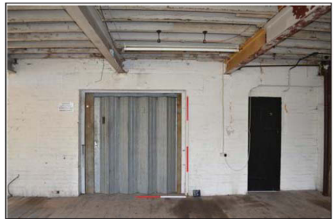
Plate 28. Room 9, Detail of goods lift, looking southwest, Scales: 2m and 1m.
