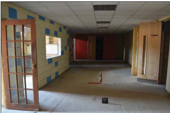
Plate 15. Room 11, general view, looking northwest, Scales: 2m and 1m.
