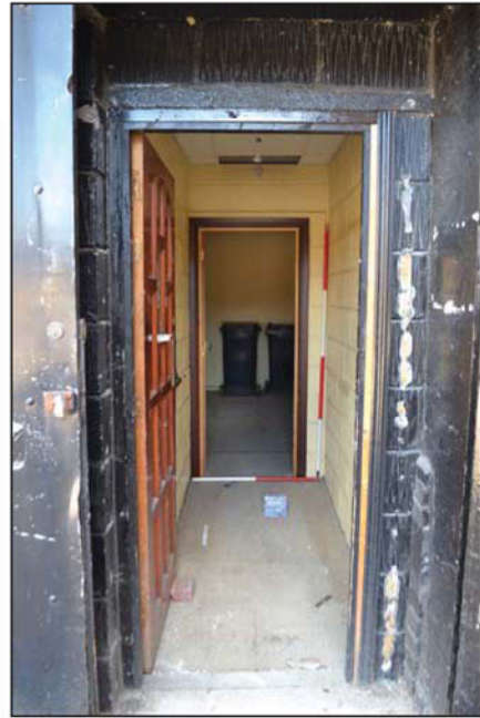
Plate 14. Entrance hallway to room 11, looking northeast, Scales: 2m and 1m.
