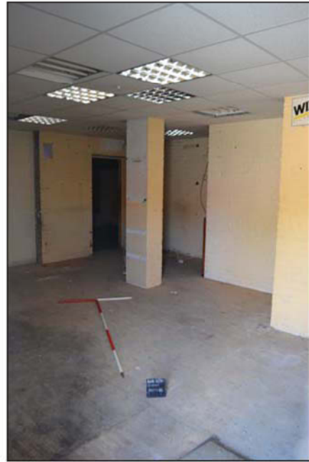
Plate 10. Room 1, view to stairs and room 2, looking east, Scales: 2m and 1m.
