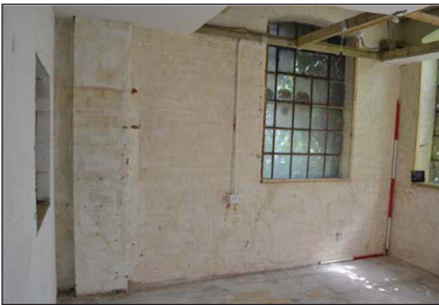
Plate 23. Room 22, Oblique view to windows, looking east, Scales: 2m and 1m.
