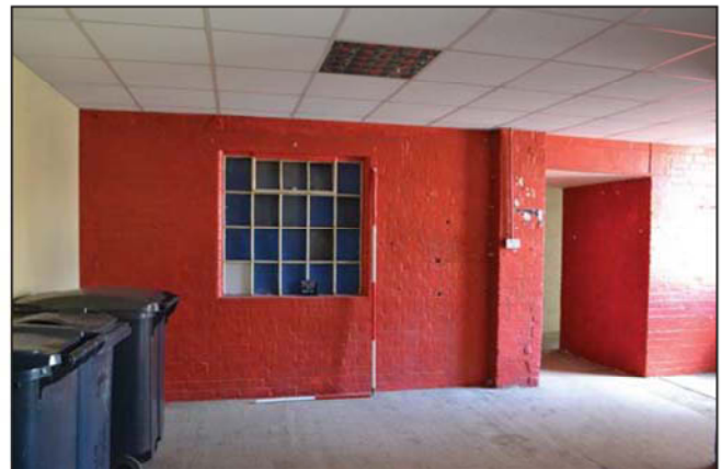
Plate 16. Room 11, former gable end window, looking southeast, Scales: 2m and 1m.
