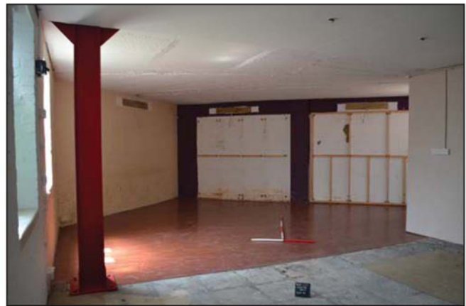
Plate 20. Room 18, general view showing steel column, looking west Scales: 2m and 1m.
