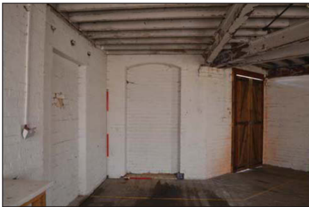
Plate 31. Room 10, Blocked door detail, looking west, Scales: 2m and 1m.
