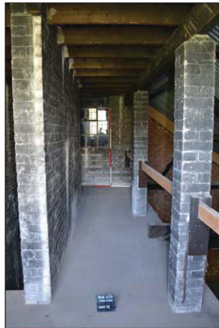
Plate 32. Stairwell, looking southwest, Scales: 2m and 1m.
