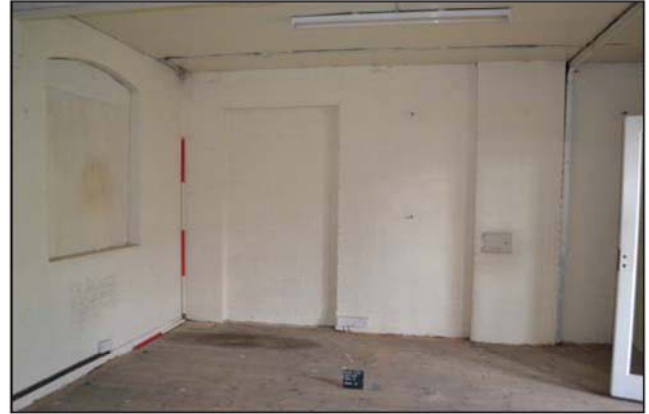
Plate 26. Room 5, View to blocked door, looking north, Scales: 2m and 1m.
