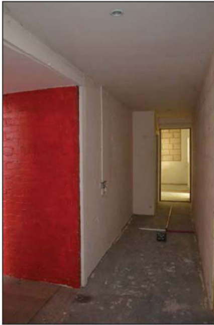
Plate 21. View along corridor, looking northeast, Scales: 2m and 1m.
