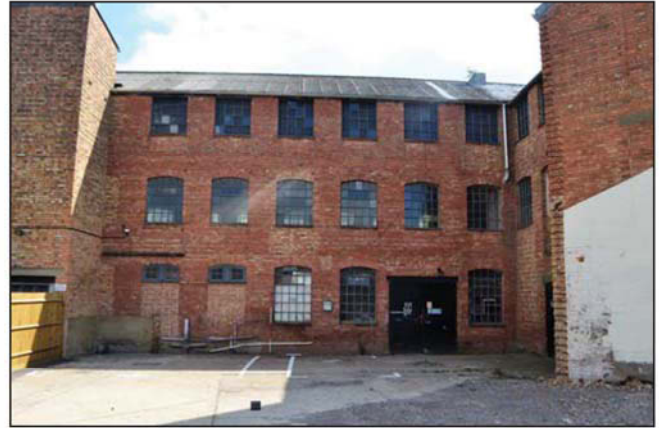
Plate 2. Exterior, original block, showing windows, looking northeast, Scales: 2m and 1m.
