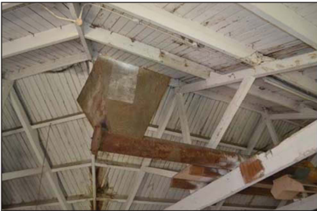
Plate 39. Room 26, Hopper in roofspace, looking northwest.
