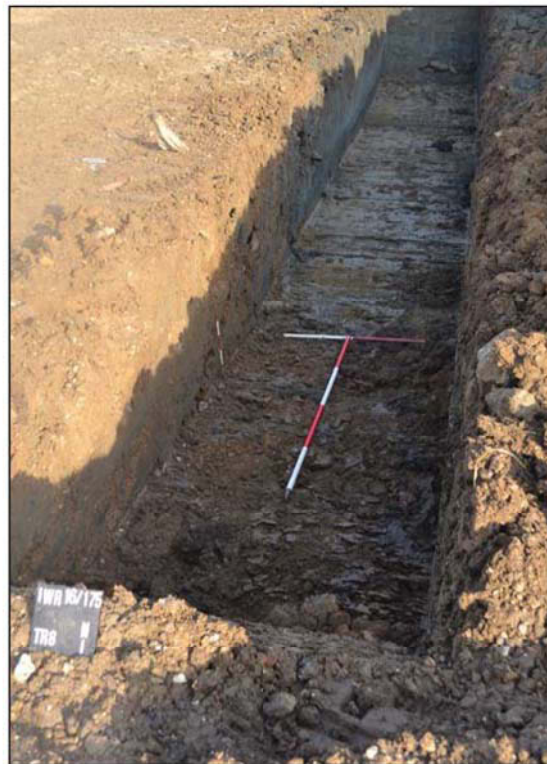
Plate 6. Trench 8, looking north, Scales: horizontal 2m and 1m, vertical 0.5m.
