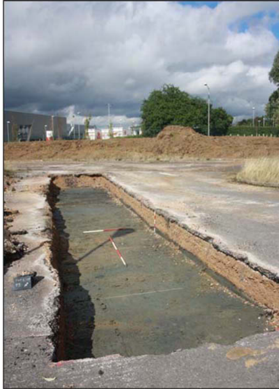
Plate 5. Trench 5, looking north west, Scales: horizontal 2m and 1m, vertical 0.5m.
