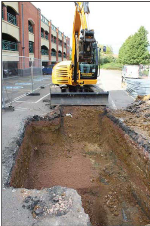
Plate 7. General setting of Trench 1, looking north.
