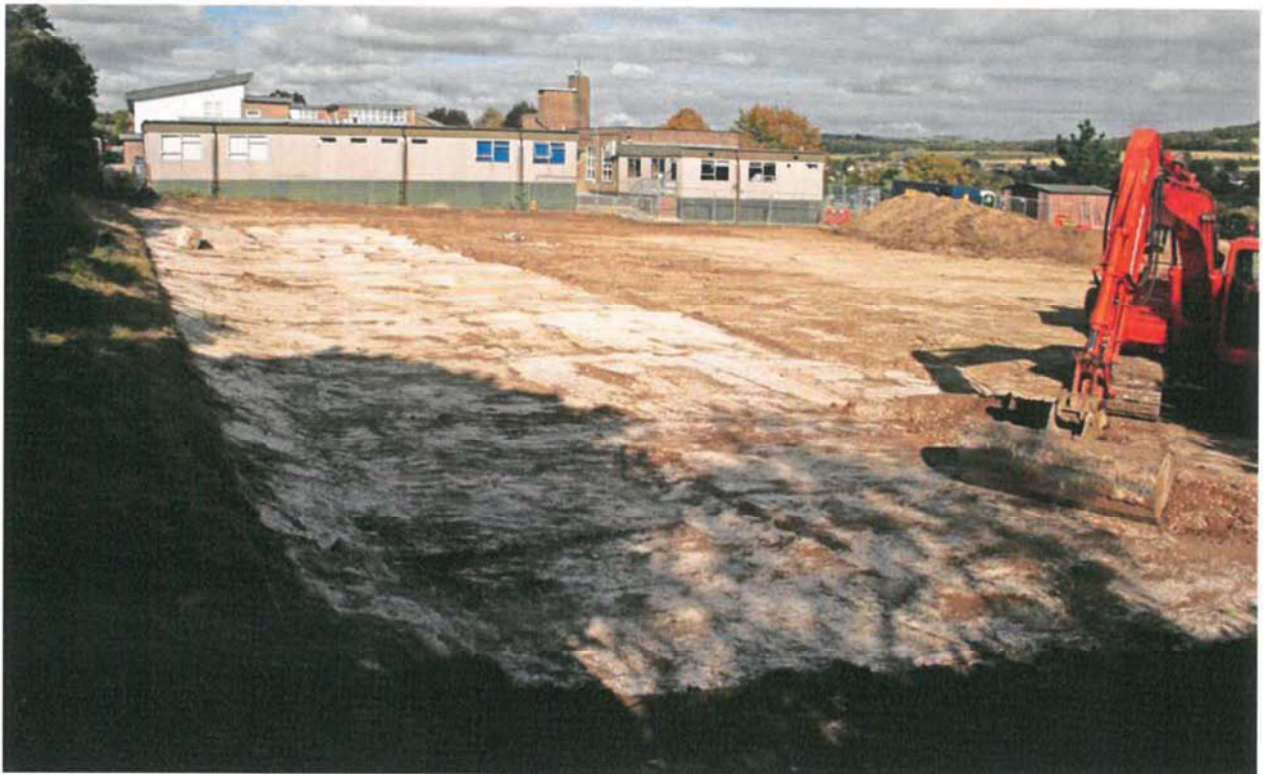
Figure 4 – West End (looking north)
