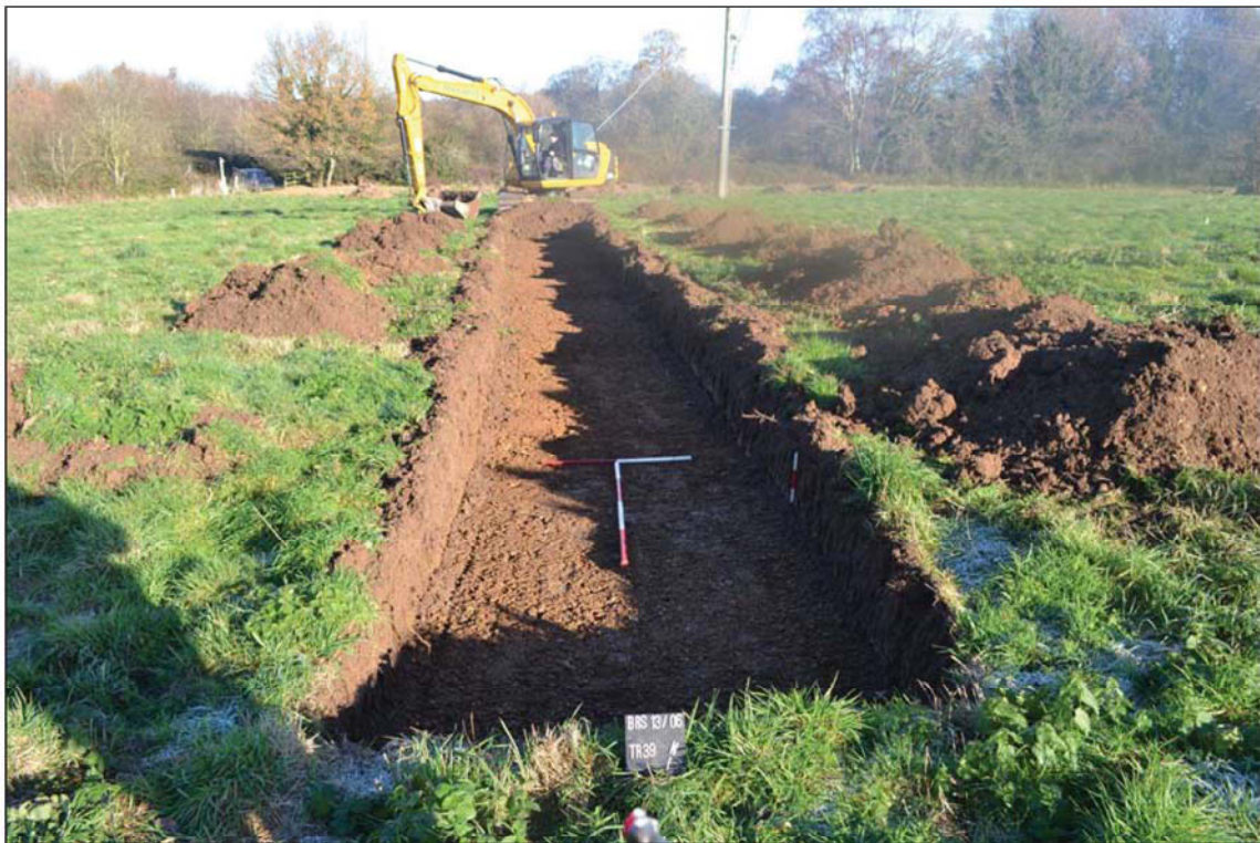
Plate 10. Trench 39, looking north west, Scales: horizontal 2m and 1m, vertical 0.3m.
