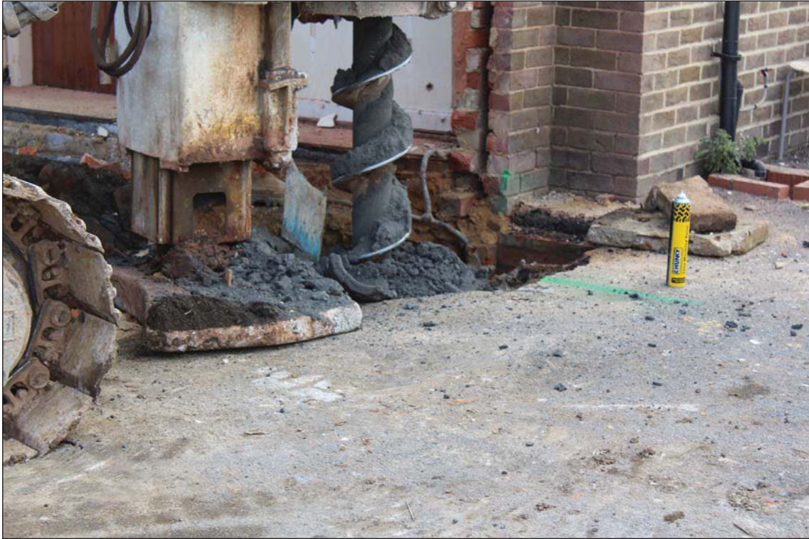
Plate 3. Piling Rig in area of Pile Hole 1
