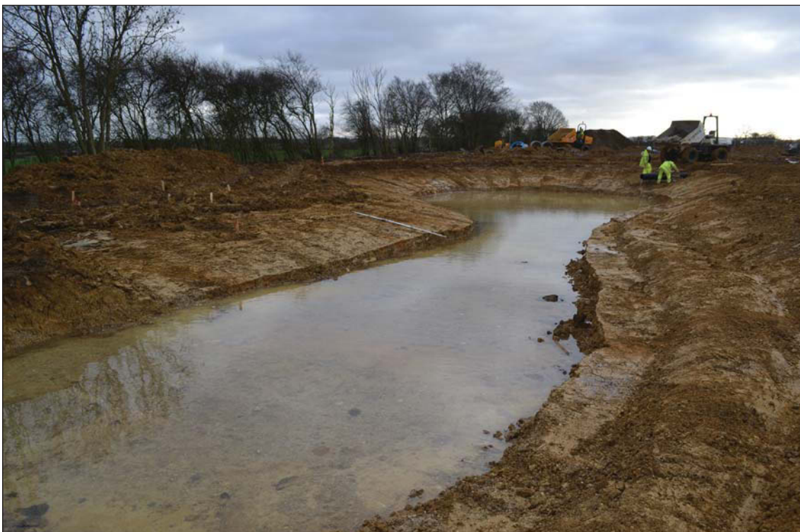
Plate 4. Grading of pond edges, looking north west.
