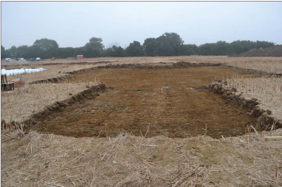
Plate 3. Topsoil strip for car parking area, looking east, Scales: 2m and 1m.
