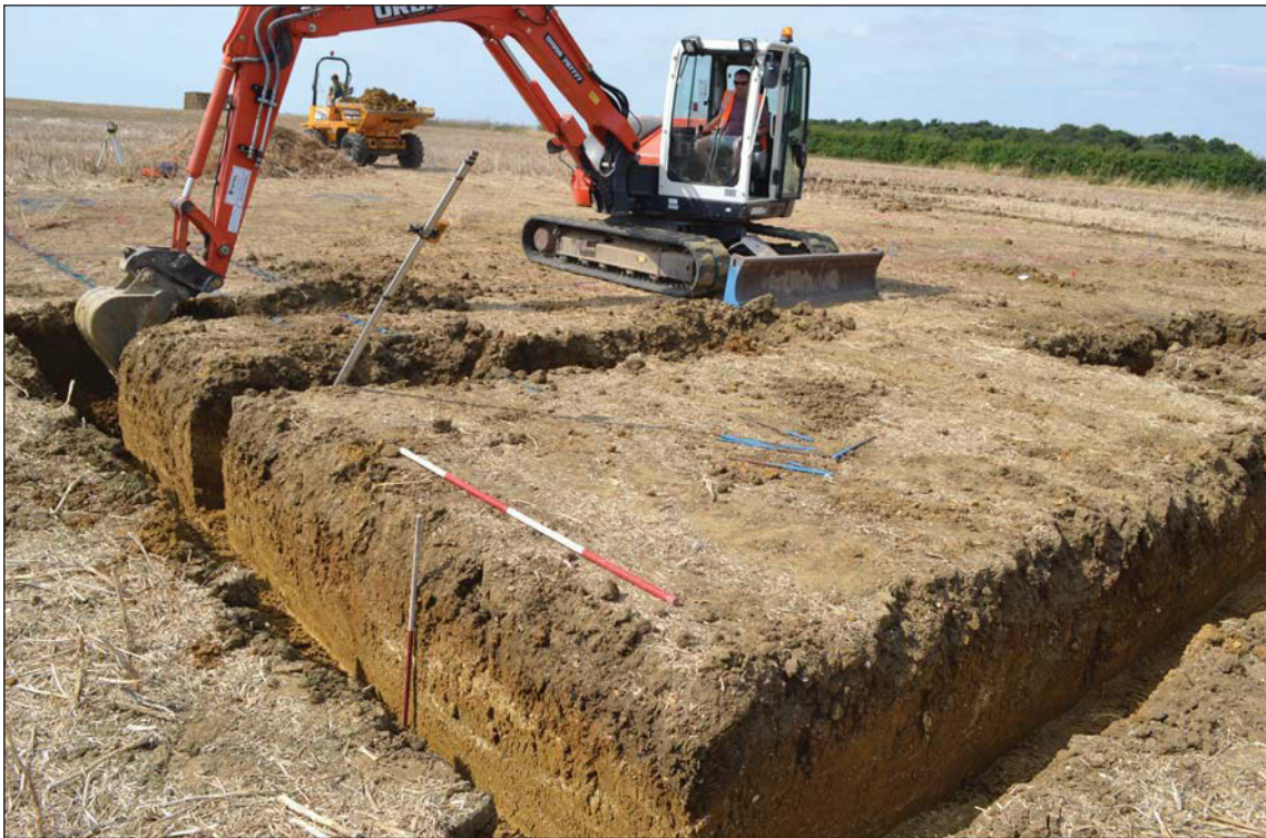
Plate 1. Footing trenches, looking north east, Scales: 2m and 1m.
