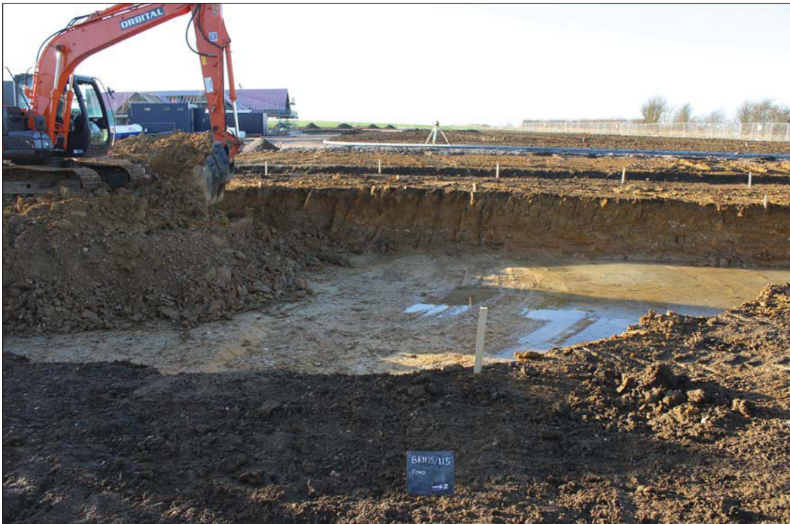
Plate 5. Full depth excavation of pond with visible section, looking west.
