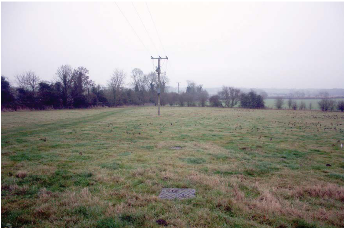
Plate 2. Site, looking ENE along the line of electric cables and manholes.
