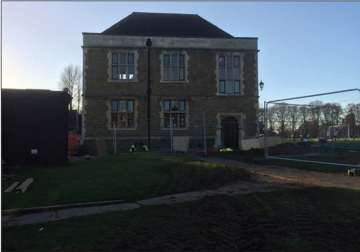
Plate 1. General view of site prior to evaluation, looking South West.
