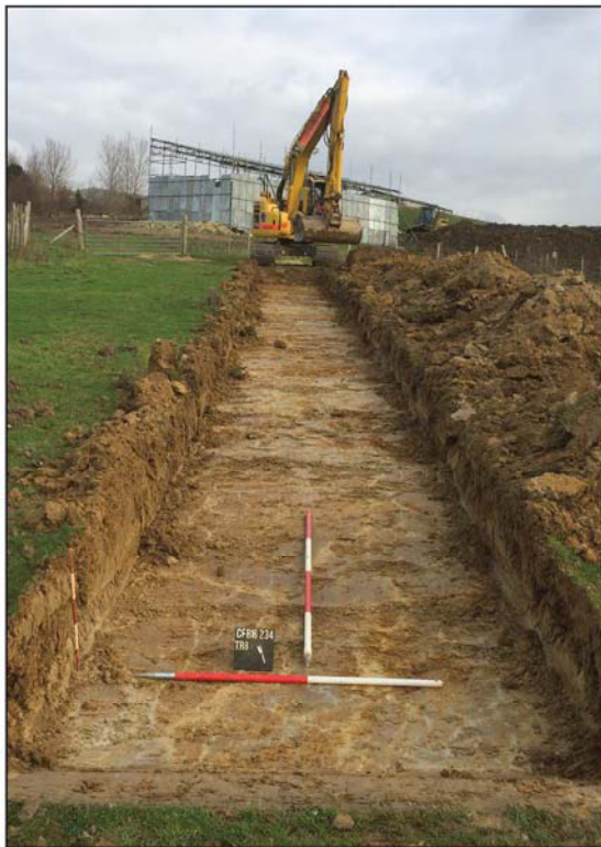
Plate 3. Trench 8, looking NE. Scales: 2m, 1m and 0.50m.
