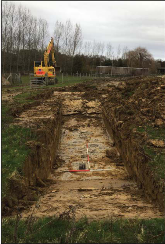
Plate 5. Trench 12, looking N. Scales: 2m, 1m and 0.50m.
