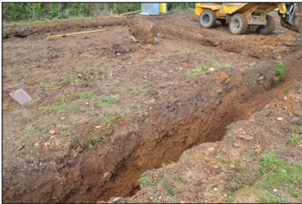
Plate 3. General view of footing trenches looking north west.
