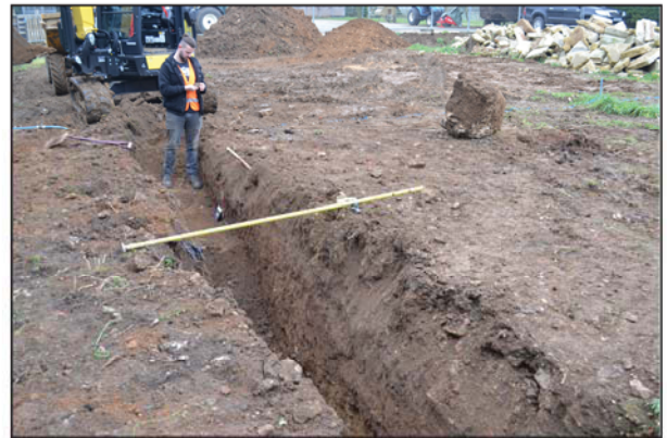
Plate 4. General view of site looking south.
