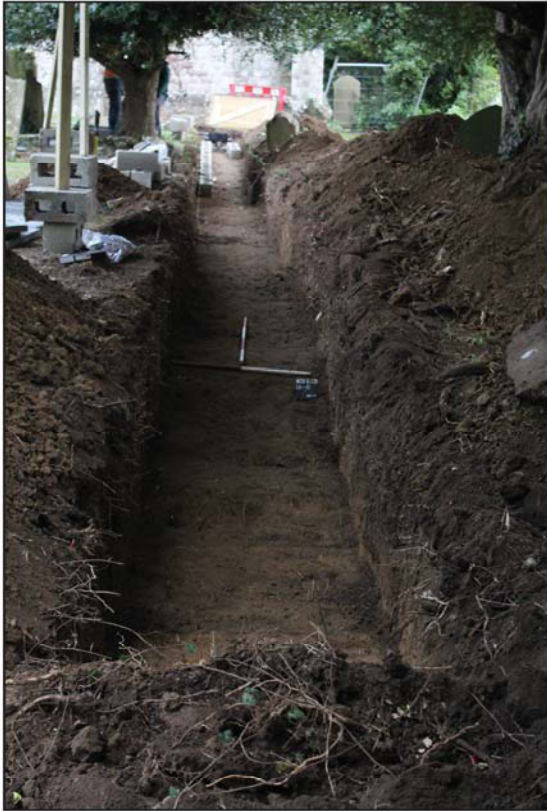
Plate 1. Drainage trench, looking East, Scales: 2m and 1m.
