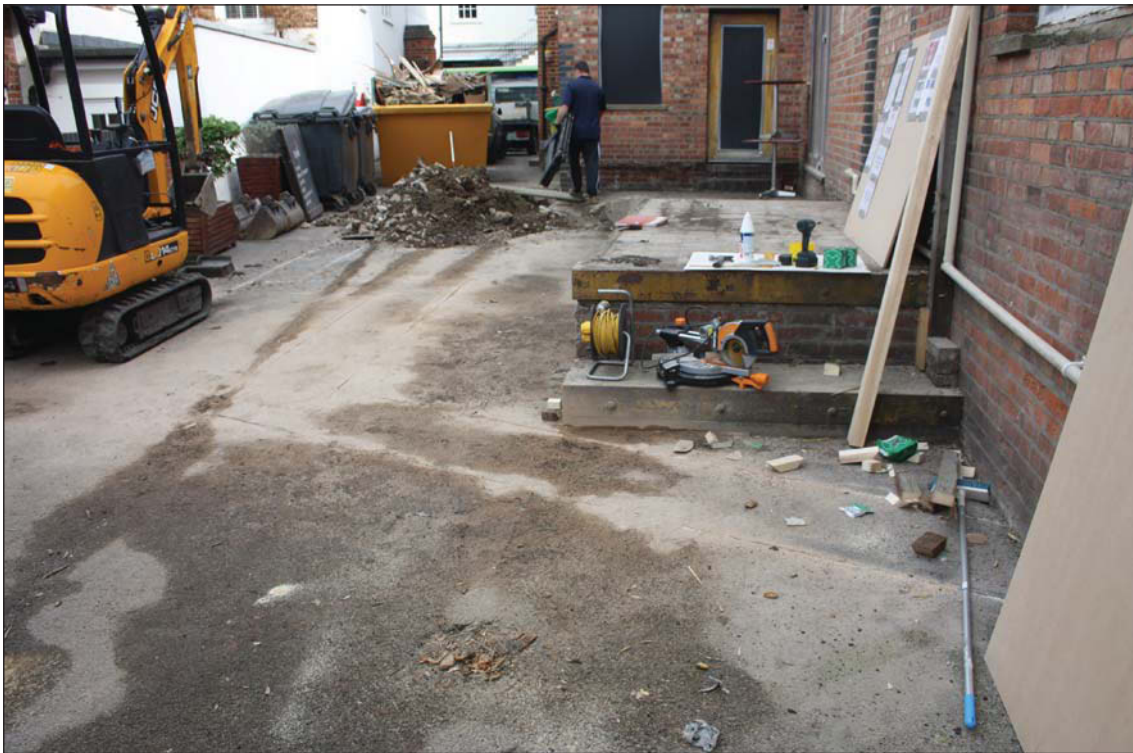
Plate 1. General view of site, looking east.
