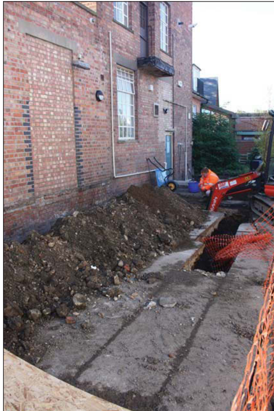
Plate 3. View of site during groundwork, looking west.
