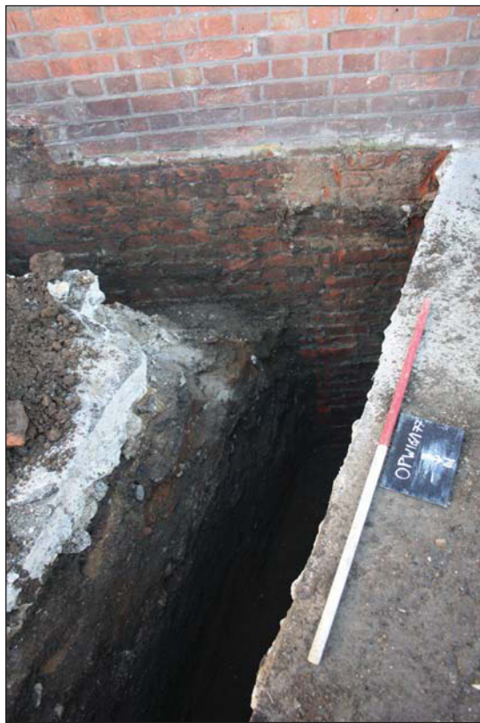
Plate 4. Deepest part of footings abutting existing wall, looking south-west, Scale: 1m.
