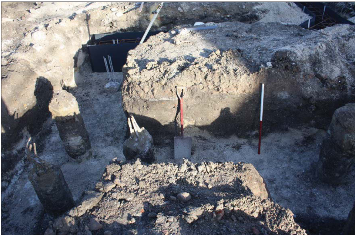
Plate 2. Footings exposing piles and section, looking north, Scale: 1m.
