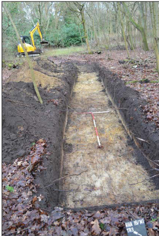
Plate 2. Trench 3, looking north-east, Scales: 2m, 1m and 0.5m.
