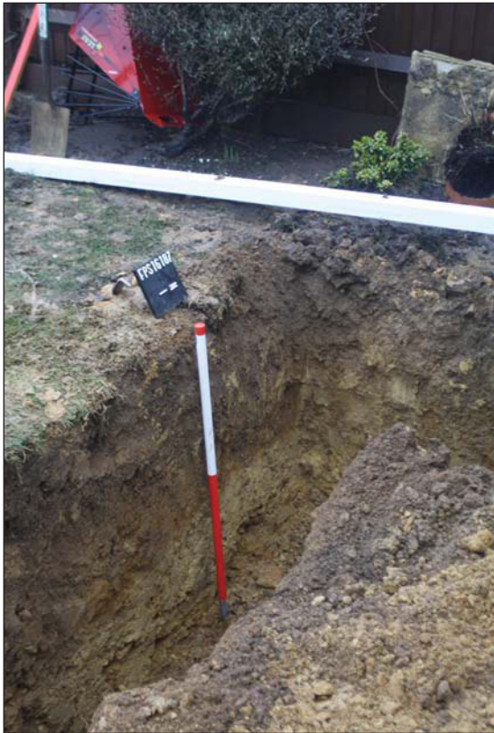
Plate 1. north-western footing trench, Looking North-West. Scale: 1m.
