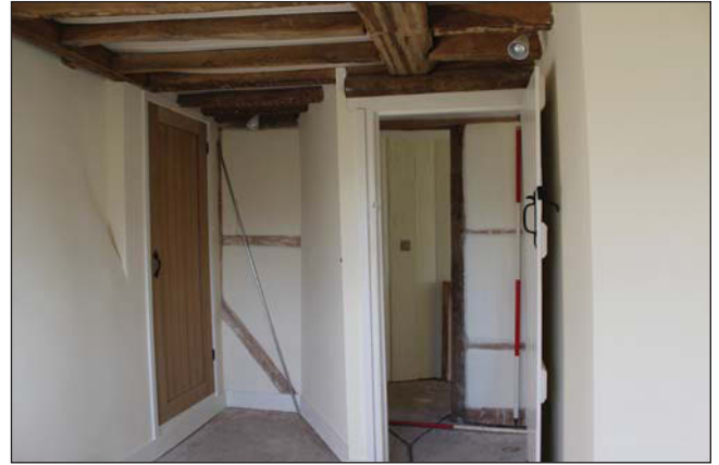
Plate 16. Internal timber framed wall, looking north-northeast, Scales: 2m and 1m.
