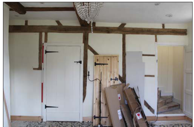
Plate 10. Internal timber framed wall, looking north-northeast, Scale: 2m.
