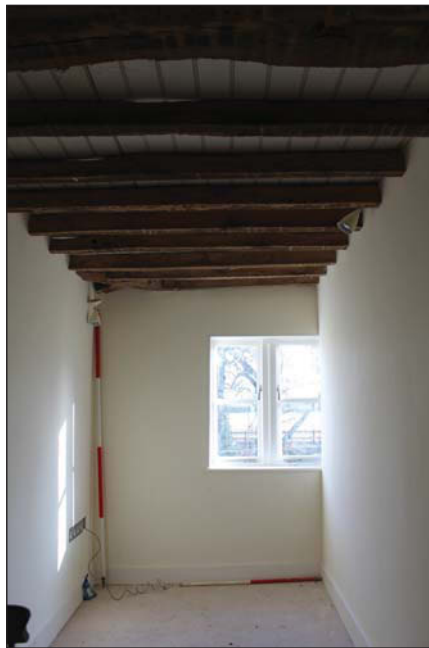
Plate 21. View to window, looking east-south-west, Scales: 2m and 1m.
