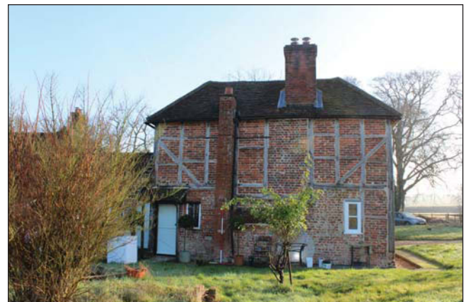
Plate 5. Rear elevation, looking east-south-east, Scales: 2m and 1m.
