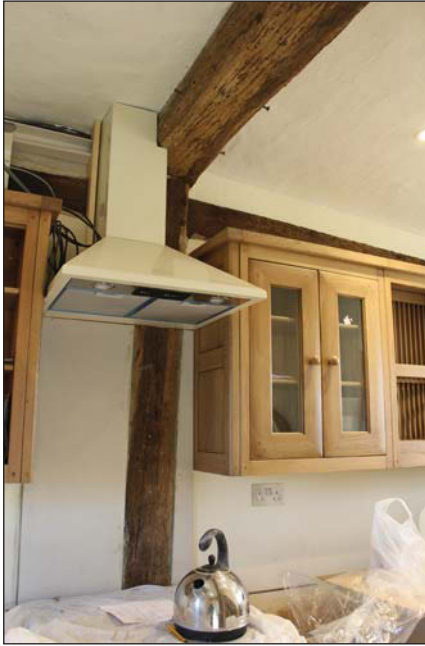
Plate 11. Timber framing within the kitchen, looking northeast.
