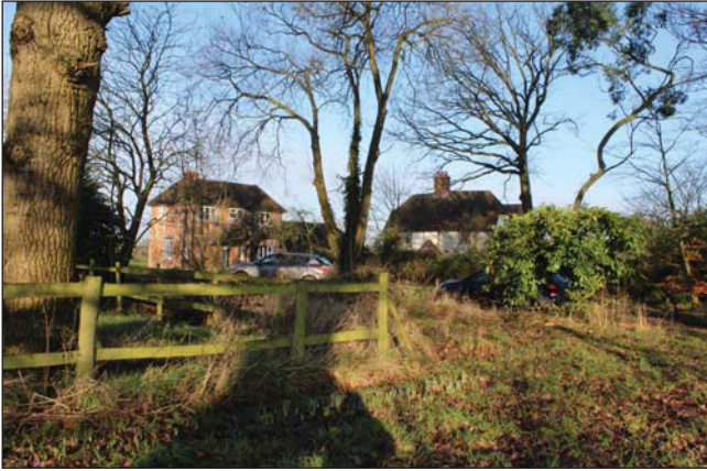
Plate 1. The Cottage and Thane Cottage, looking north west.
