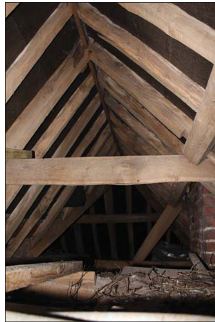
Plate 22. Roof detail, looking east.
