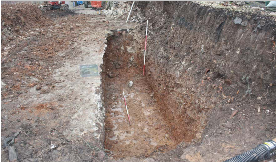
Plate 2. Retaining wall trench, looking north, Scales: 2m, and 2m
